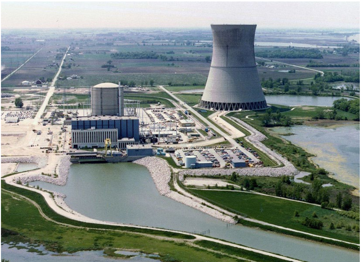
Davis-Besse nuclear plant in northern Ohio | NRC
