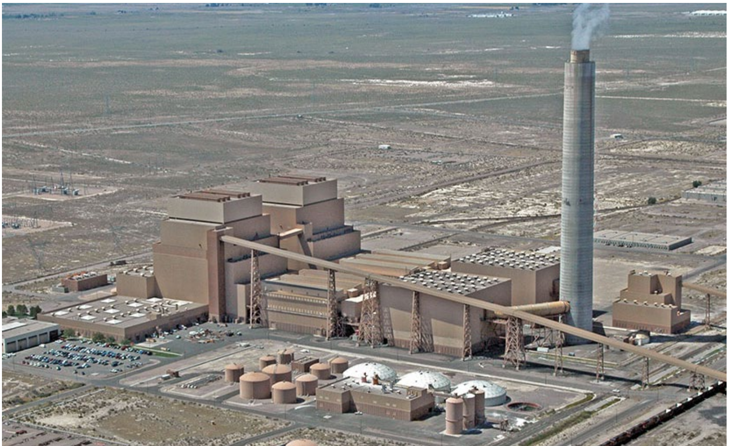
LADWP plans to convert the coal-fired Intermountain Power Plant in Utah into the first electricity generating plant capable of burning a large portion of hydrogen in its fuel mix, starting with 30% in 2025 and eventually rising to 100%. | Green Hydrogen Coalition
