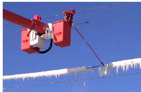
A lineman clears ice from transmission lines. | MISO
