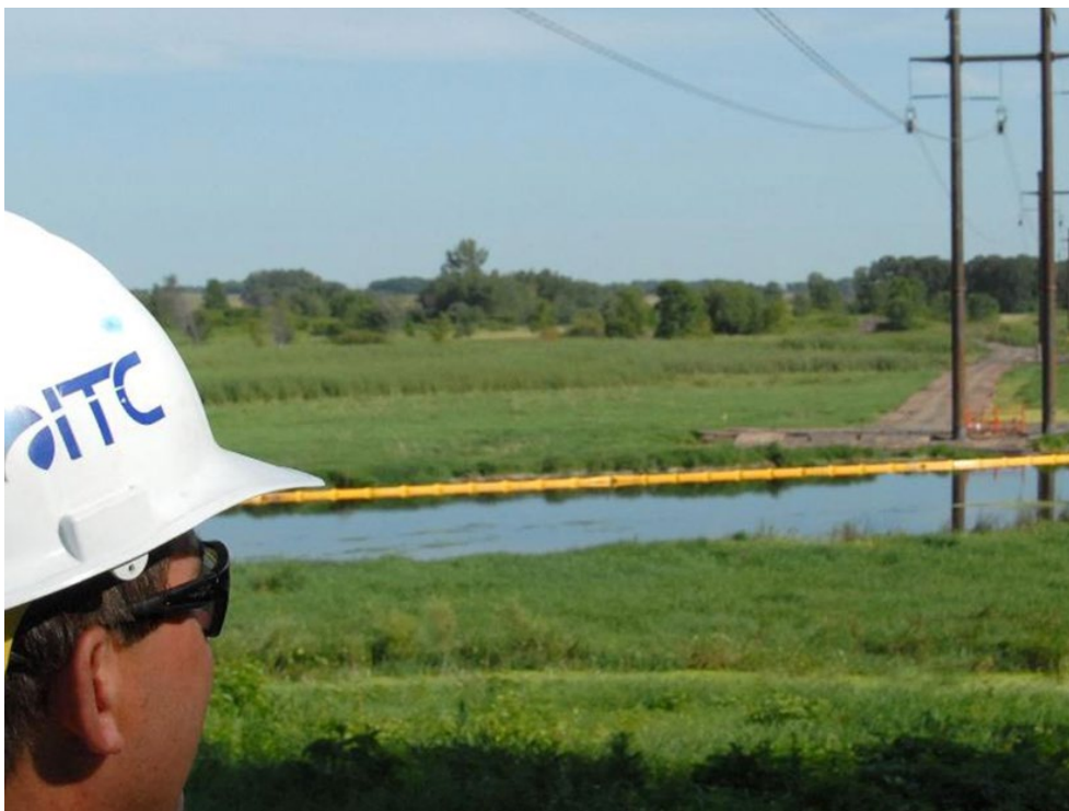
ITC Holdings calls itself the largest independent electric transmission company in the U.S., with projects in operation or under development in Michigan, Iowa, Minnesota, Illinois, Missouri, Kansas, Oklahoma and Wisconsin. | ITC Holdings
