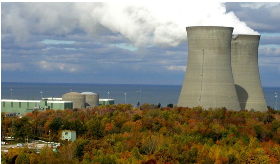
The Perry nuclear plant in Ohio | Nuclear Regulatory Commission
