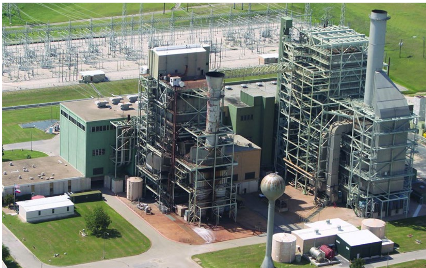
Decker Creek Power Station | Austin Energy
