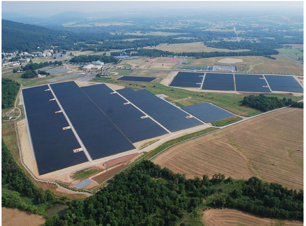
Utility Scale Solar in Maryland | Constellation
