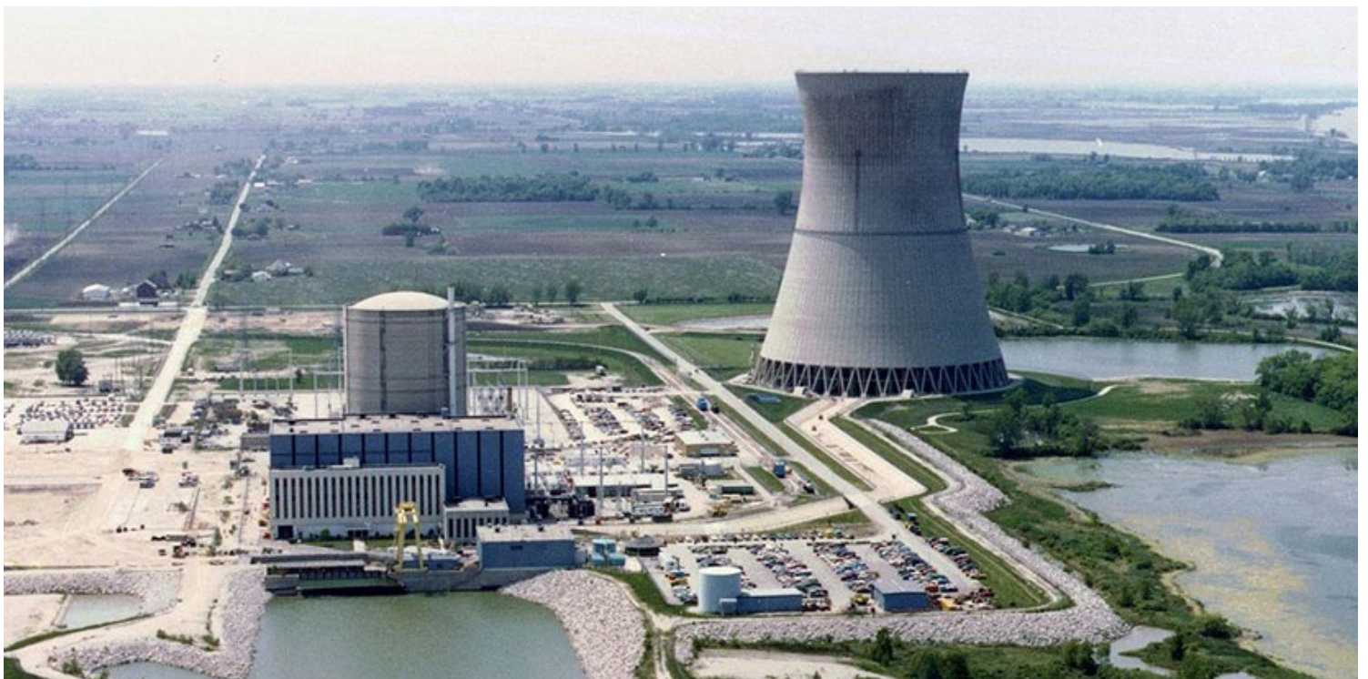
Davis-Besse nuclear plant in northern Ohio | NRC
