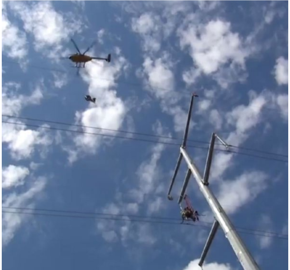
Ameren Illinois line work | Ameren Illinois
