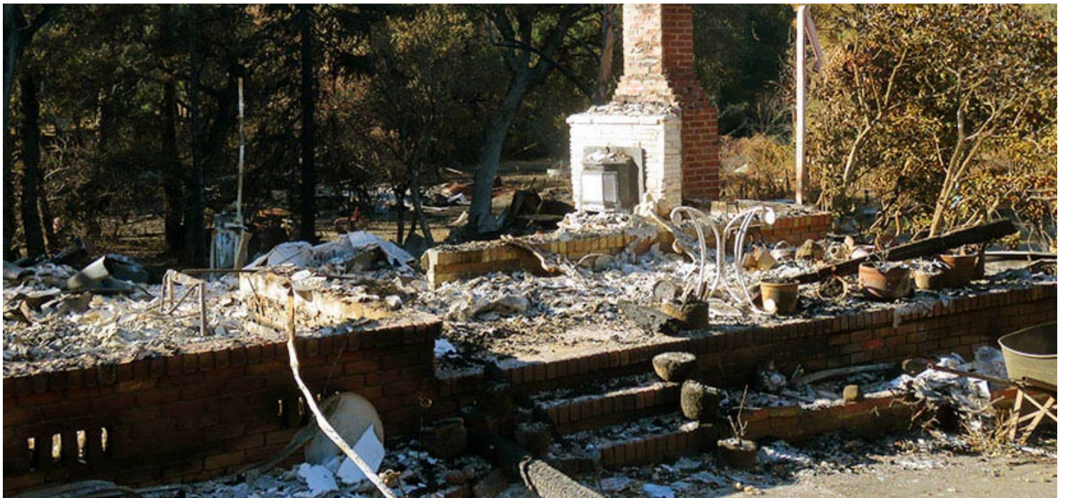
One of the 174 homes in Sonoma County destroyed by the Kincadee Fire in October 2019 | © RTO Insider LLC
