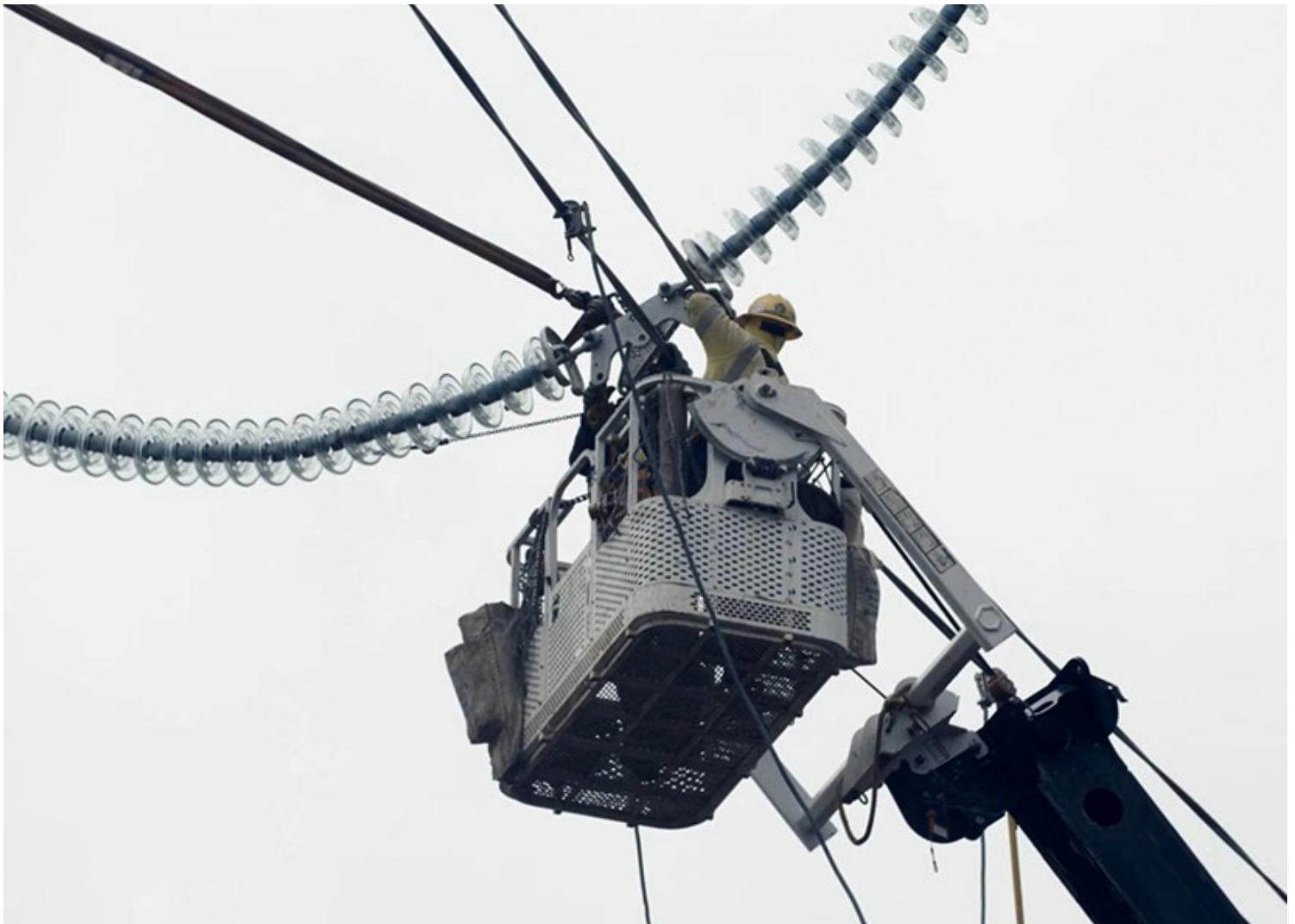
Construction of the MISO MVP Badger - Coulee line in Wisconsin | IBEW
