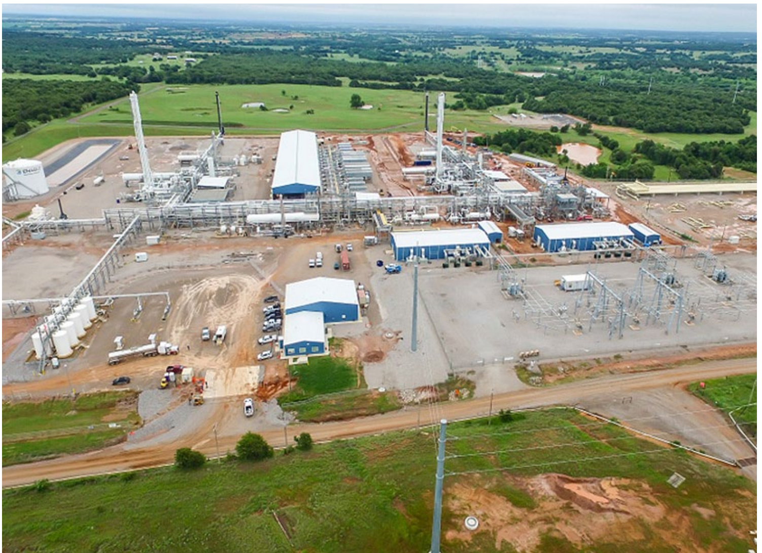
Enable Midstream Partners processing plant | Enable
