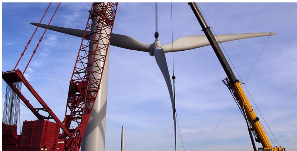
Construction at an Invenergy wind facility | Invenergy
