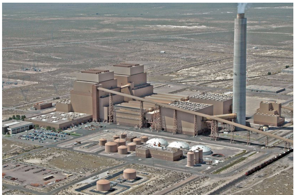
Intermountain Power Plant in Delta, Utah, which LADWP plans to convert from coal to a gas-fired plant capable of burning a fuel mixture containing green hydrogen. | Green Hydrogen Coalition
