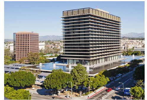
LADWP headquarters | LADWP
