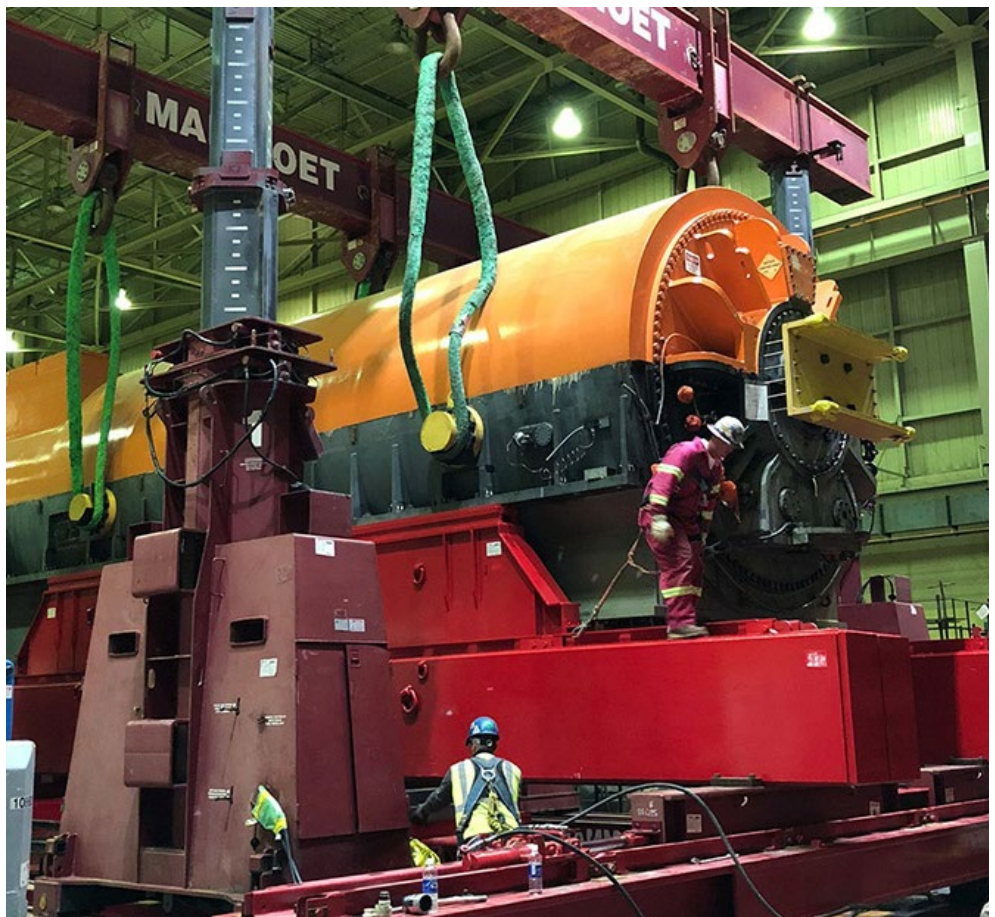
Work at an Xcel Energy nuclear power station | Xcel Energy
