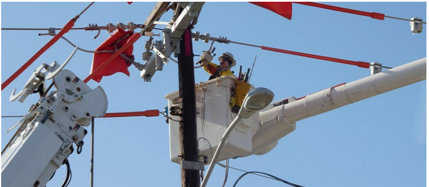
Line work in AEP's Southwestern Electric Power Co. territory | SWEPCO
