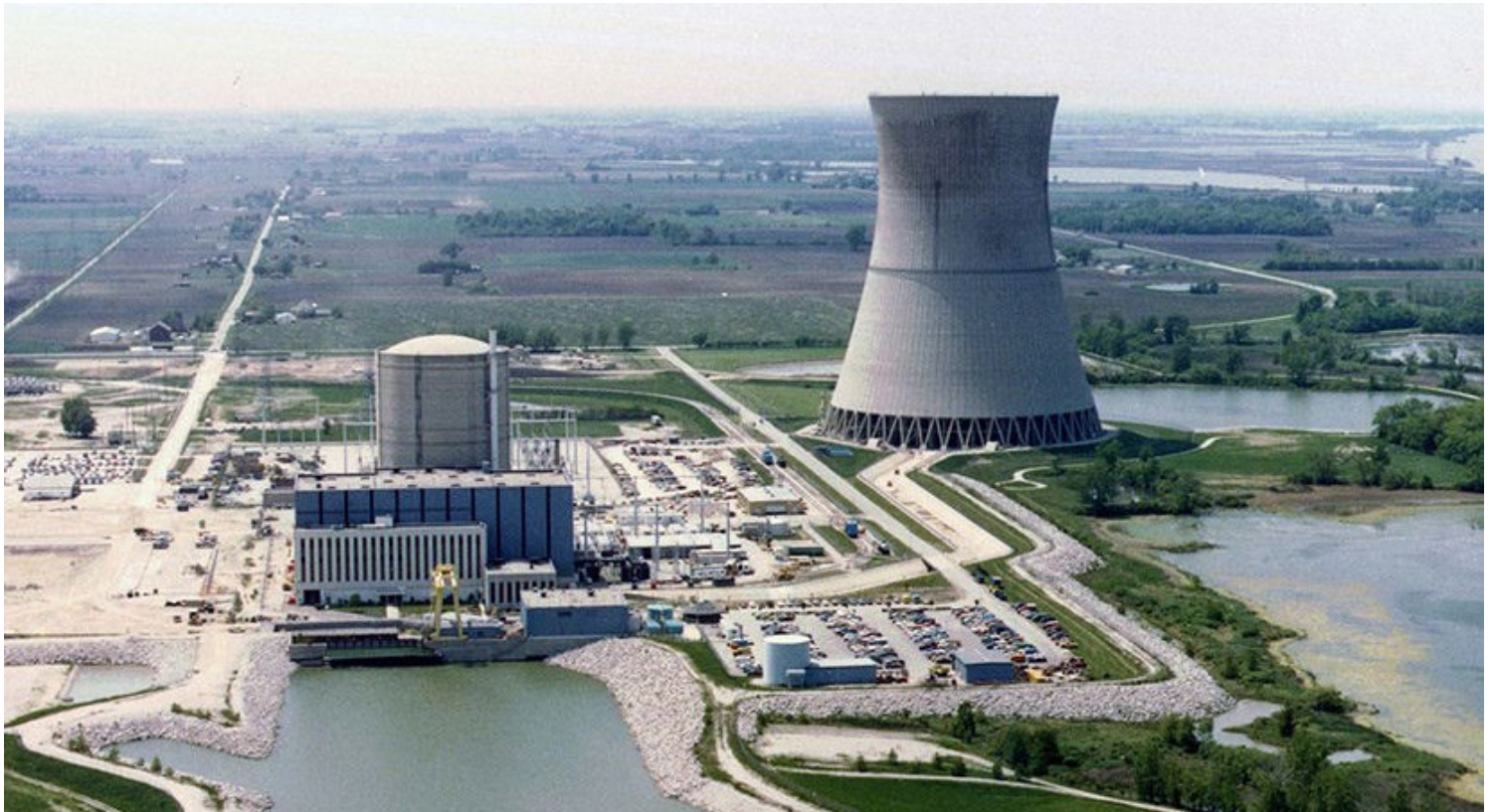
Davis-Besse nuclear plant in northern Ohio | NRC
