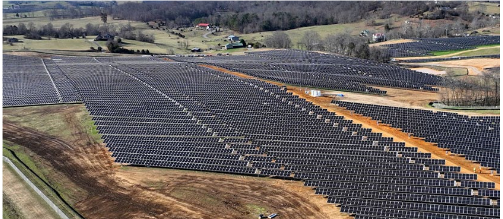
TVA and BrightRidge's new Martin Solar Farm in east Tennessee | TVA
