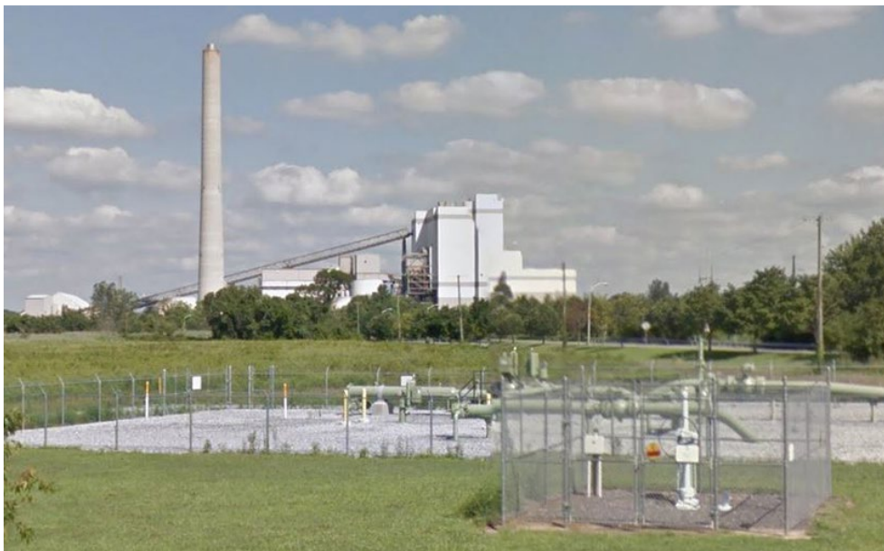
Logan Generating Plant | Google Maps
