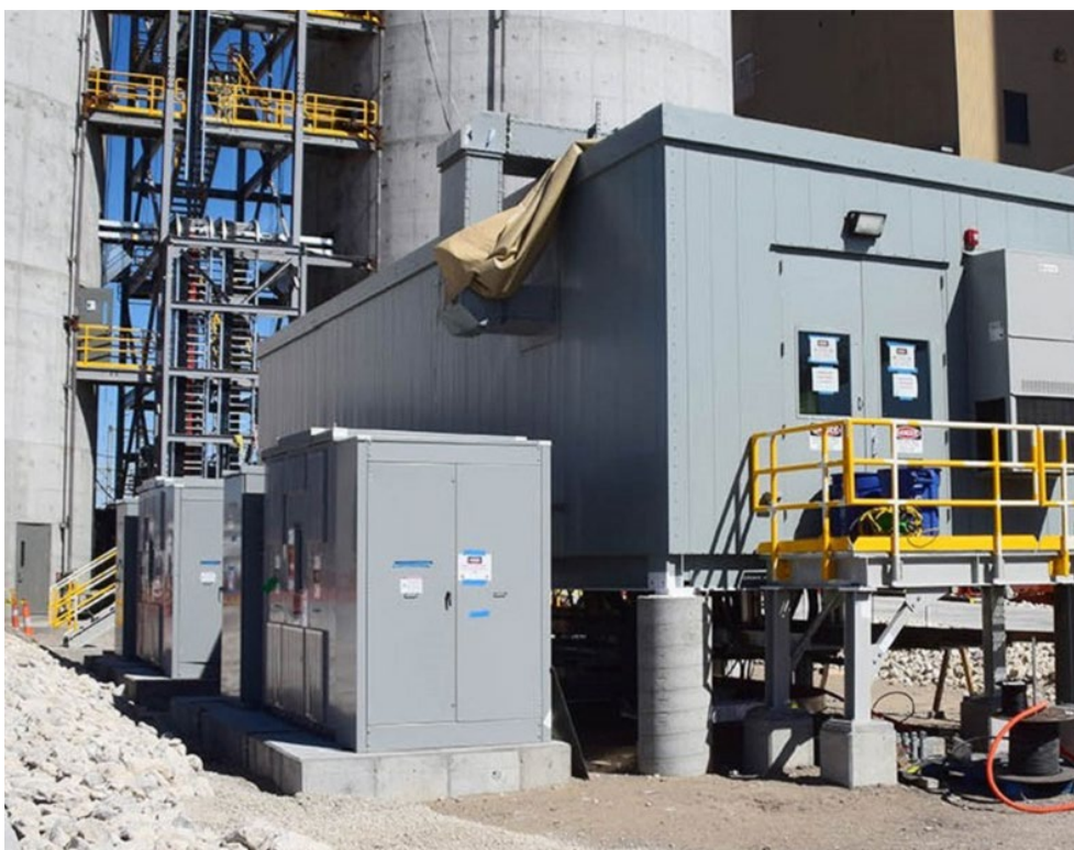
Upgrade work at Rush Island Energy Center in 2018 | McCarthy Construction
