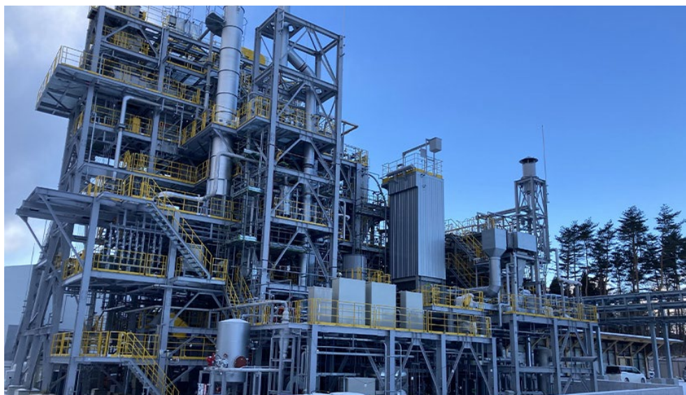
Carbon capture technology from LanzaTech converts solid waste to ethanol at a Japanese chemical plant. | Sekisui
