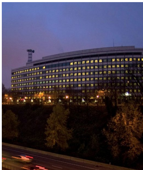
BPA headquarters in Portland, Ore. | DOE
