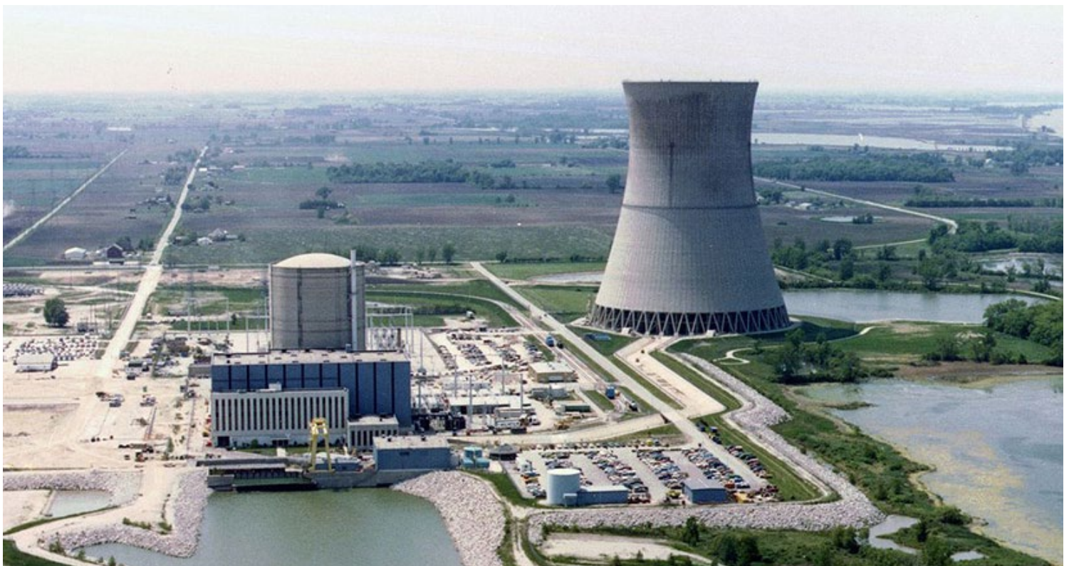
Davis-Besse nuclear plant in northern Ohio | NRC
