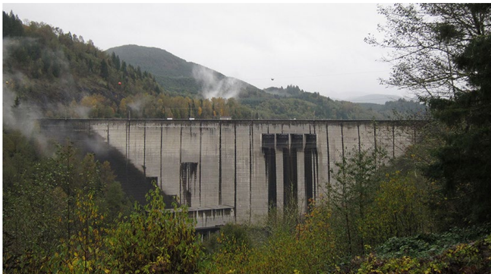
Tacoma Power's Mossyrock Dam is part of the Cowlitz River Project, one of four hydroelectric projects operated by the municipal utility. | Jaywm, CC BY-SA 4.0, via Wikimedia
