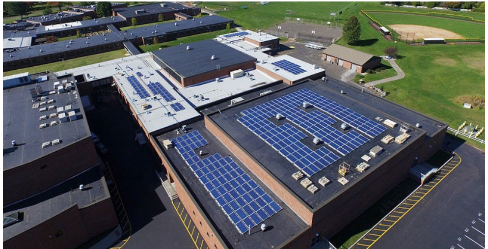
An 876-kW solar installation in Hopewell, N.J. | Advanced Solar Products
