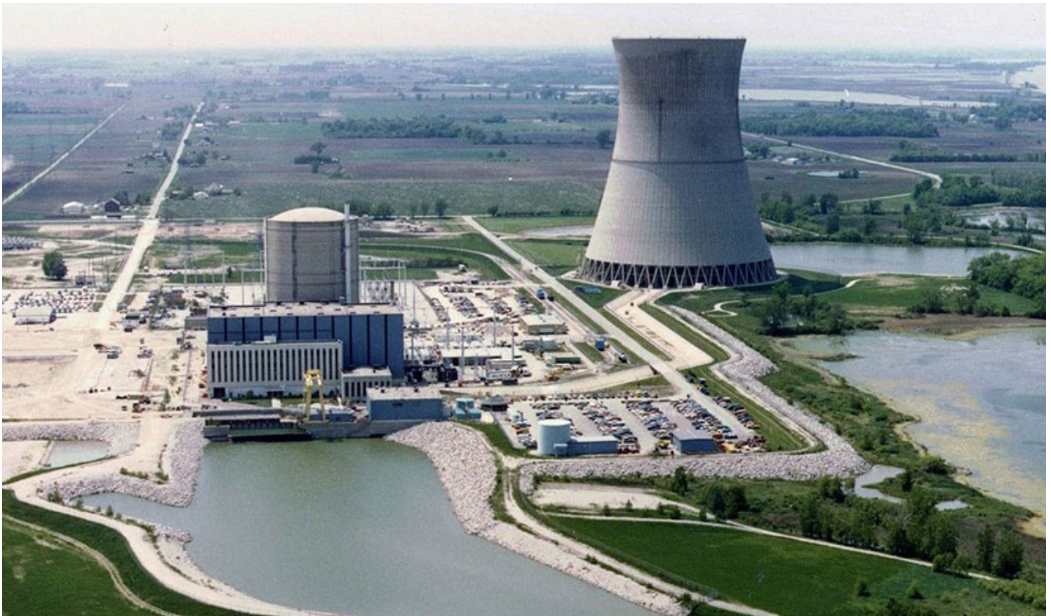
Davis-Besse nuclear plant in northern Ohio | NRC
