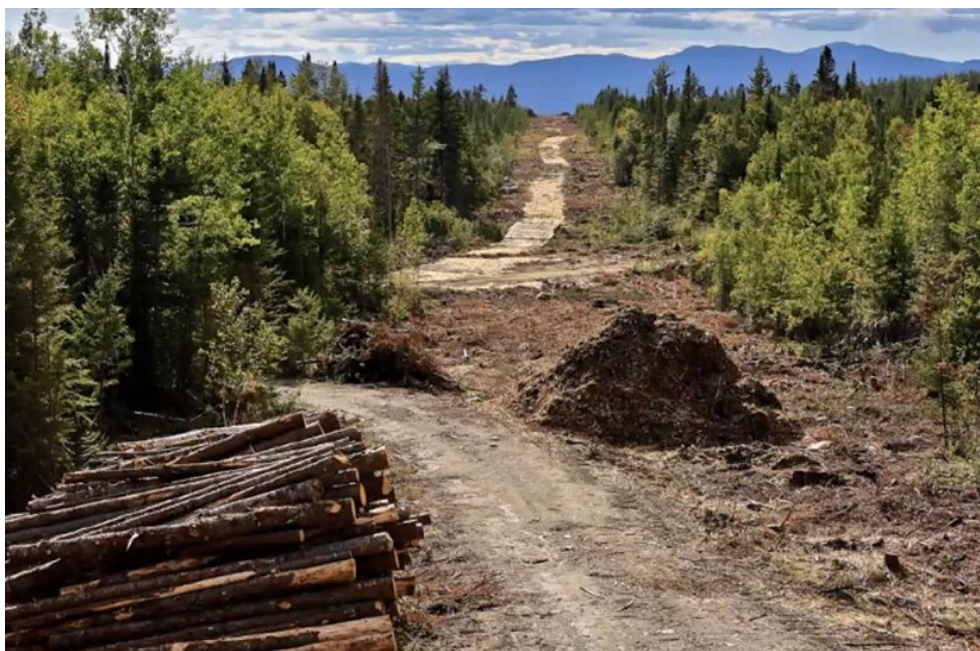
The fate of the New England Clean Energy Connect transmission line should serve as a warning about future projects, said Maine PUC Chair Phil Bartlett. | Roger Merchant
