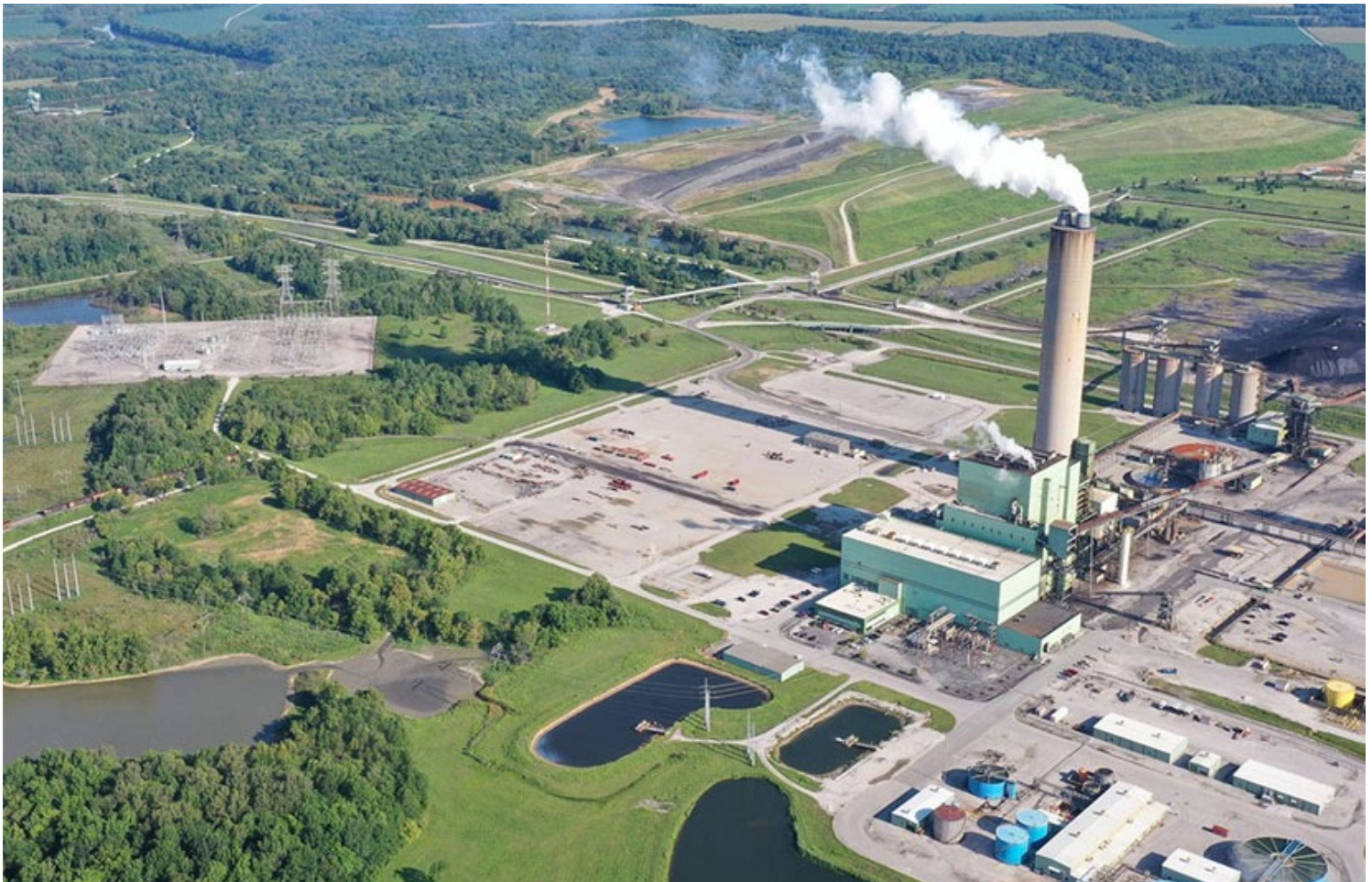
DB Wilson Station | Big Rivers Electric Corp.
