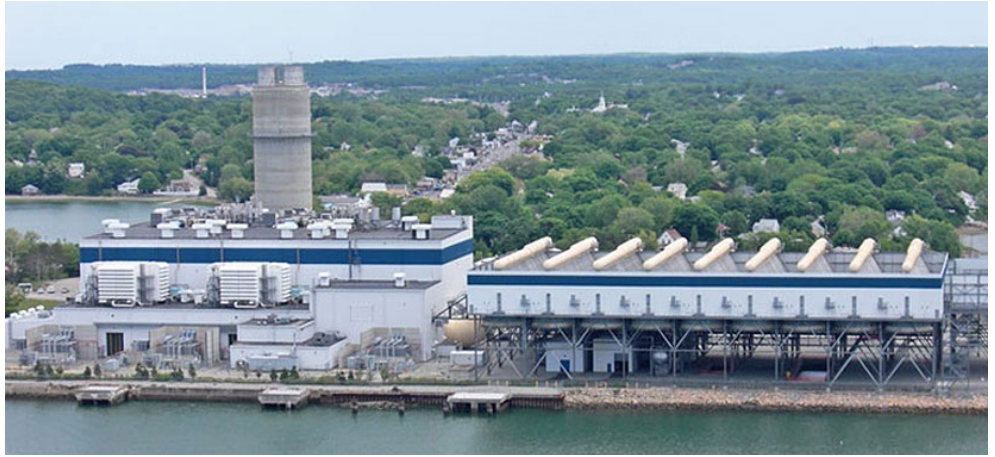
Fore River Energy Center in Weymouth, Mass. | Calpine
