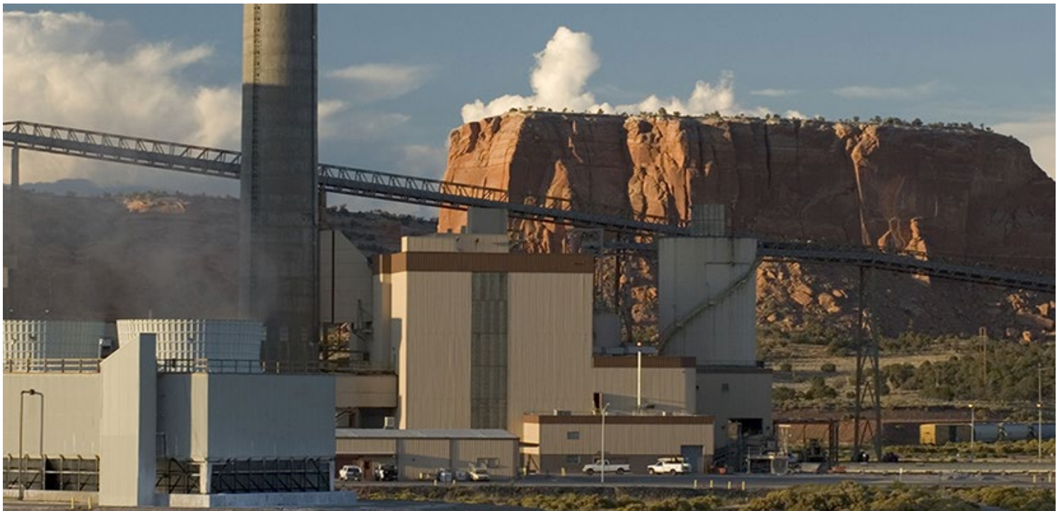
Coal plant belonging to Tri-State Generation and Transmission, one of a number of utilities and marketers that endorsed the motion urging FERC to extend the cost justification filing deadline to 30 days. | Tri-State Generation and Transmission
