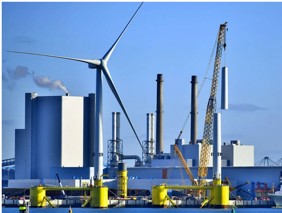
Assembling floating wind turbines for the West Coast will require large port facilities, like those in Rotterdam used for Scotland's Kincardine Offshore Windfarm. | Principle Power
