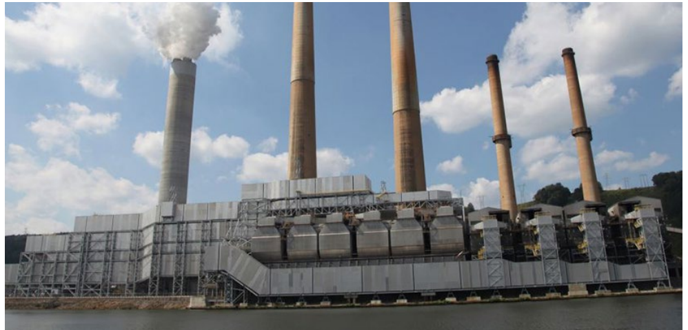
Energy Harbor’s 1,504.3-MW W.H. Sammis Power Station at Stratton, Ohio, is set to be deactivated in 2023. | FirstEnergy Solutions
