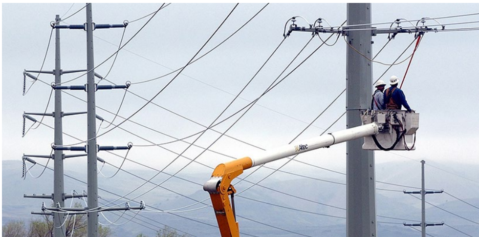
Lineworkers on PacifiCorp transmission line | PacifiCorp
