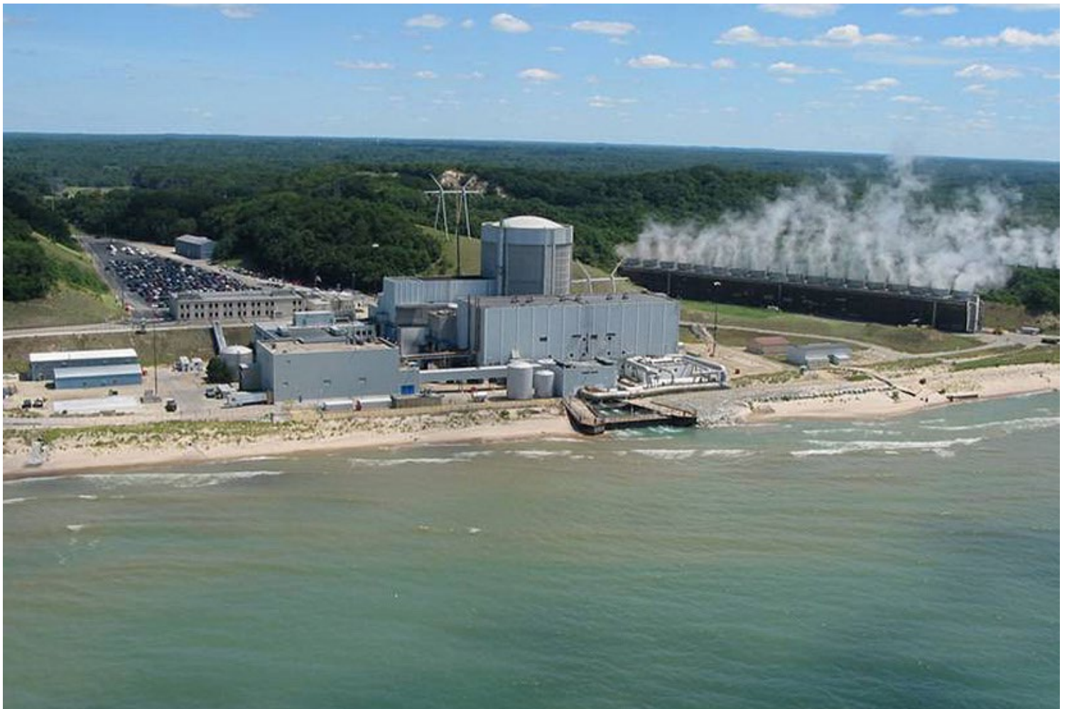
The Palisades nuclear plant | Nuclear Regulatory Commission
