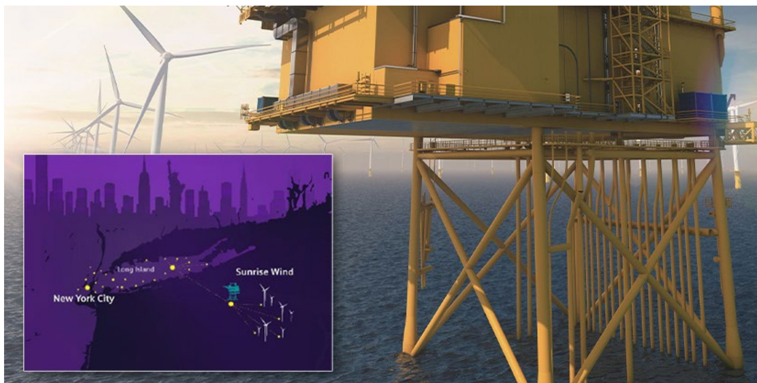
The offshore converter station will collect the alternating current power generated by Sunrise Wind's turbines and transform it to direct current. | Siemens Energy
