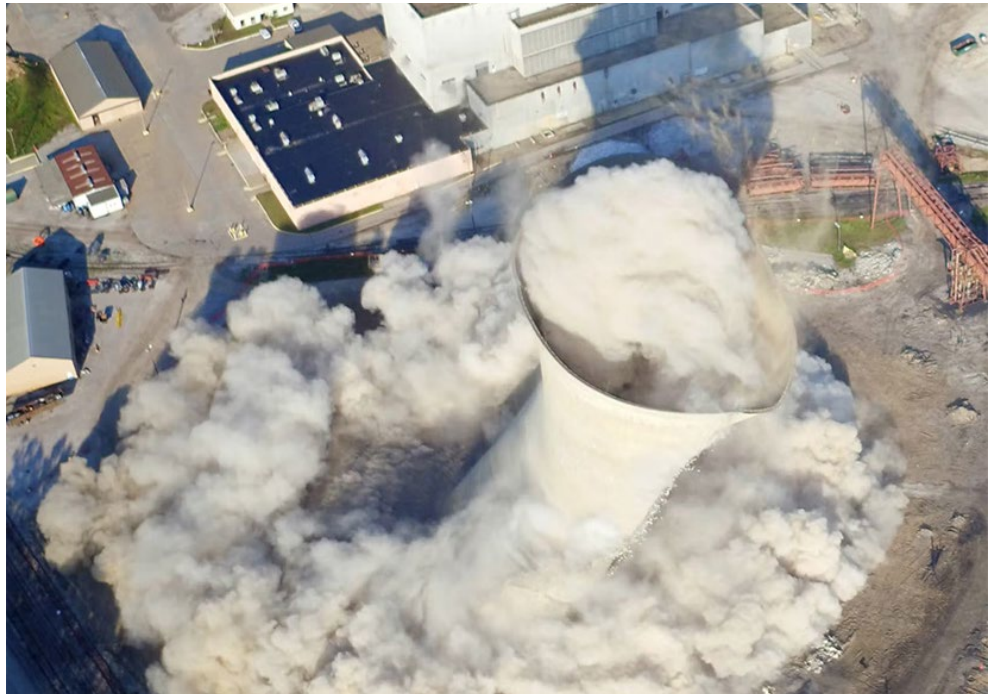
Implosion of a Big Sandy cooling tower in 2016 | Independence Demolition
