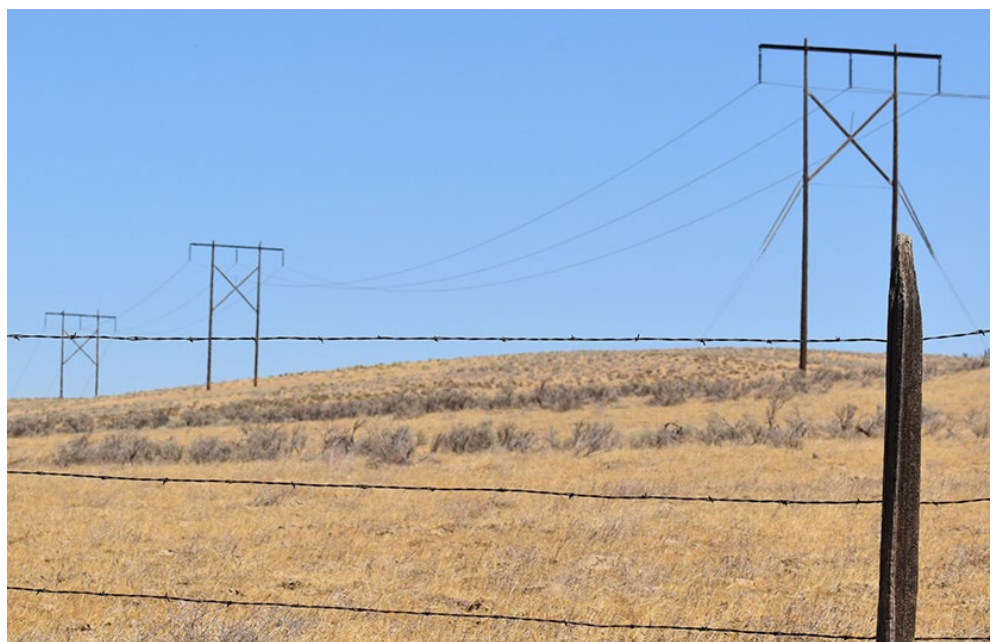
Transmission line in Umatilla County, Ore. | © RTO Insider LLC
