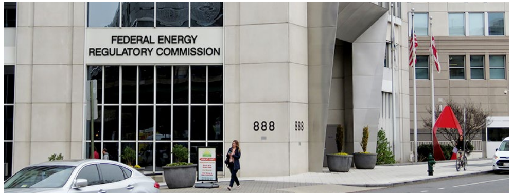
FERC headquarters in D.C. | © RTO Insider LLC
