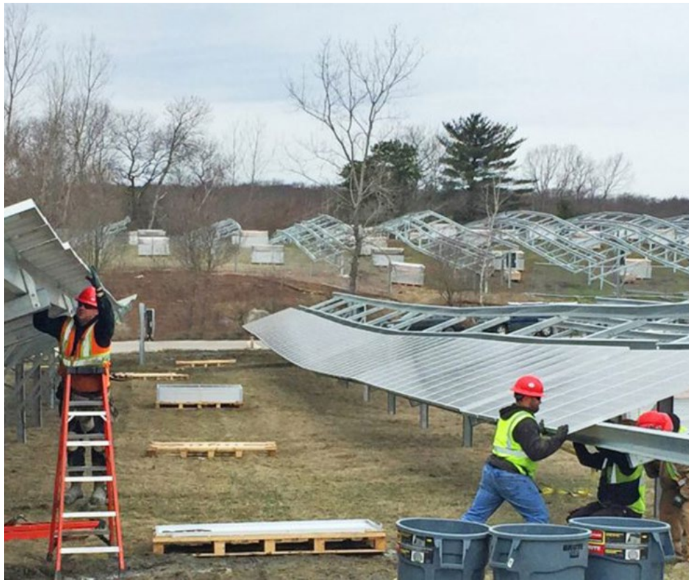
Utility scale solar project under construction | CS Energy
