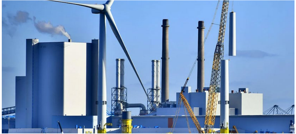
Assembling floating wind turbines for the West Coast will require large port facilities, like those in Rotterdam used for Scotland's Kincardine Offshore Windfarm. | Principle Power
