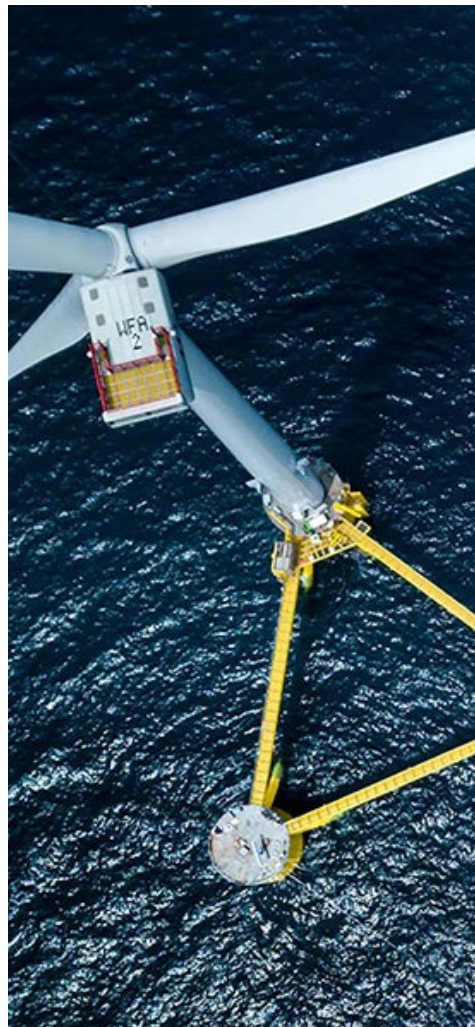
Wind power off the coast of California will require floating platforms because of ocean depths. | Principle Power
