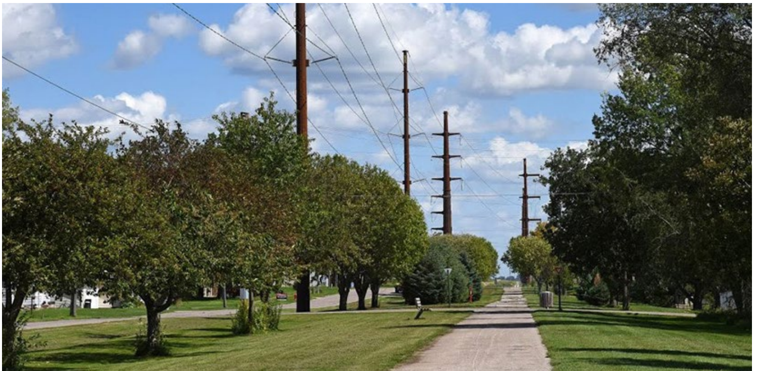
ITC Midwest's Traer-Dysart 161-kV line in Iowa | ITC Holdings
