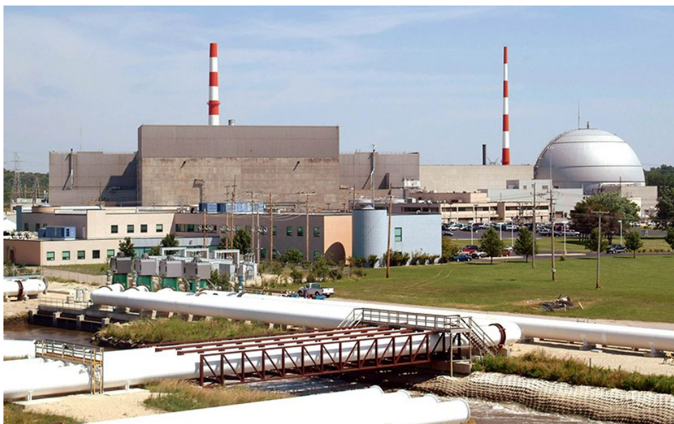
All of Constellation Energy's 16,175 MW of nuclear capacity cleared in PJM's 2023/24 capacity auction, including the Byron, Dresden (pictured) and Quad Cities plants in Illinois, which were left out of the money last year. | American Nuclear Society
