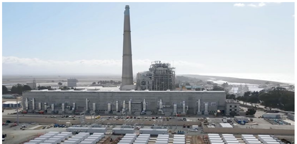
The addition of large amounts of storage resources, such as PG&E's 182.5-MW Elkhorn Battery project, is one reason for the CPUC's new RA framework. | EKM Metering
