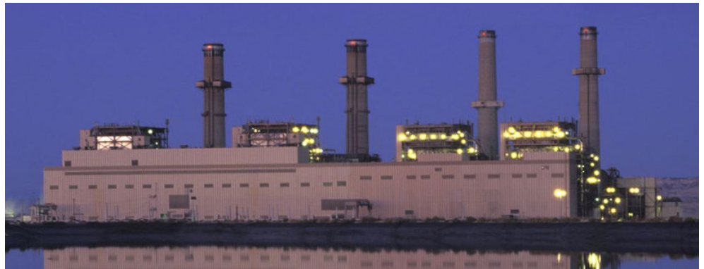
San Juan Generating Station | PNM
