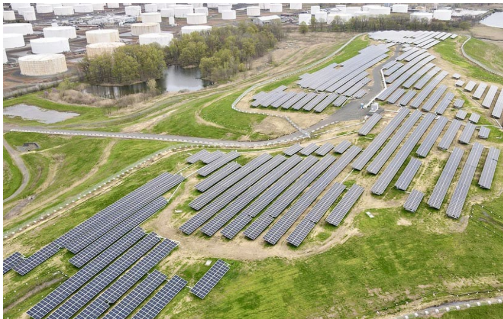
Navisun's 4.5-MW Linden Hawk Rise community solar project, located on a former landfill site in Linden, N.J. | Navisun
