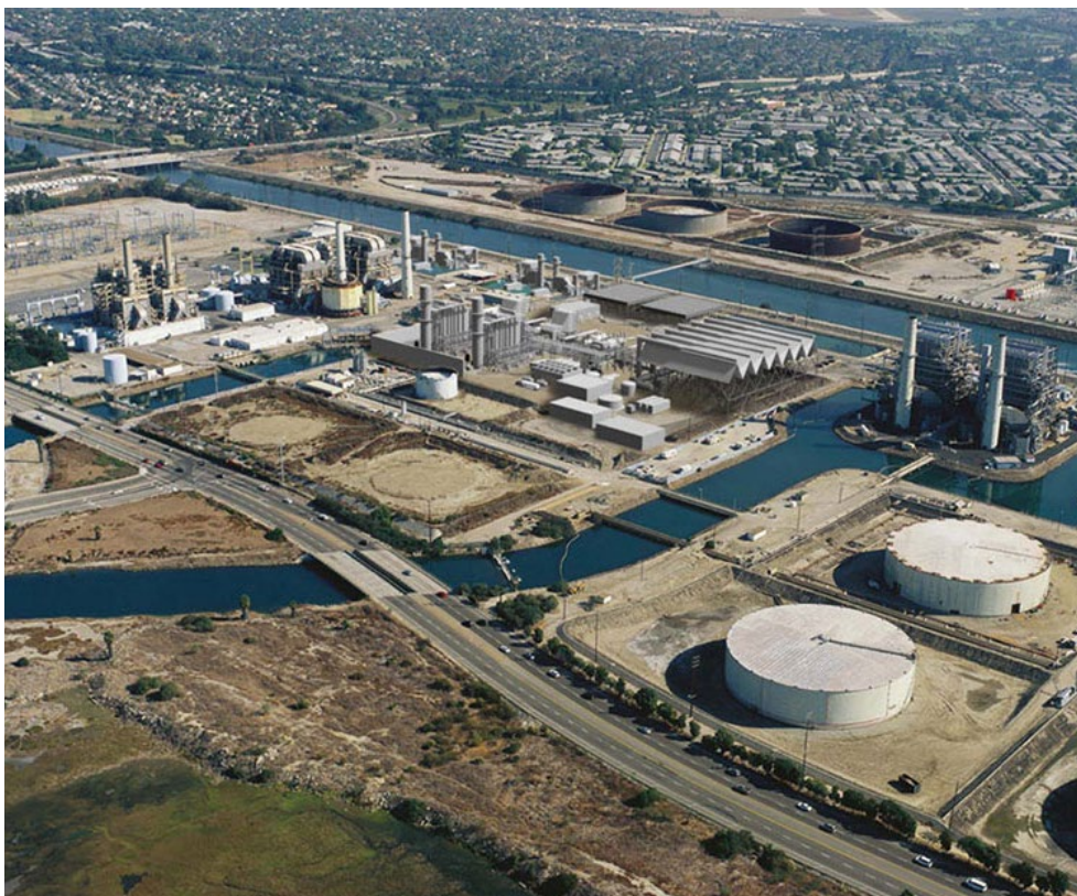
Alamos Generating Station | California Energy Commission
