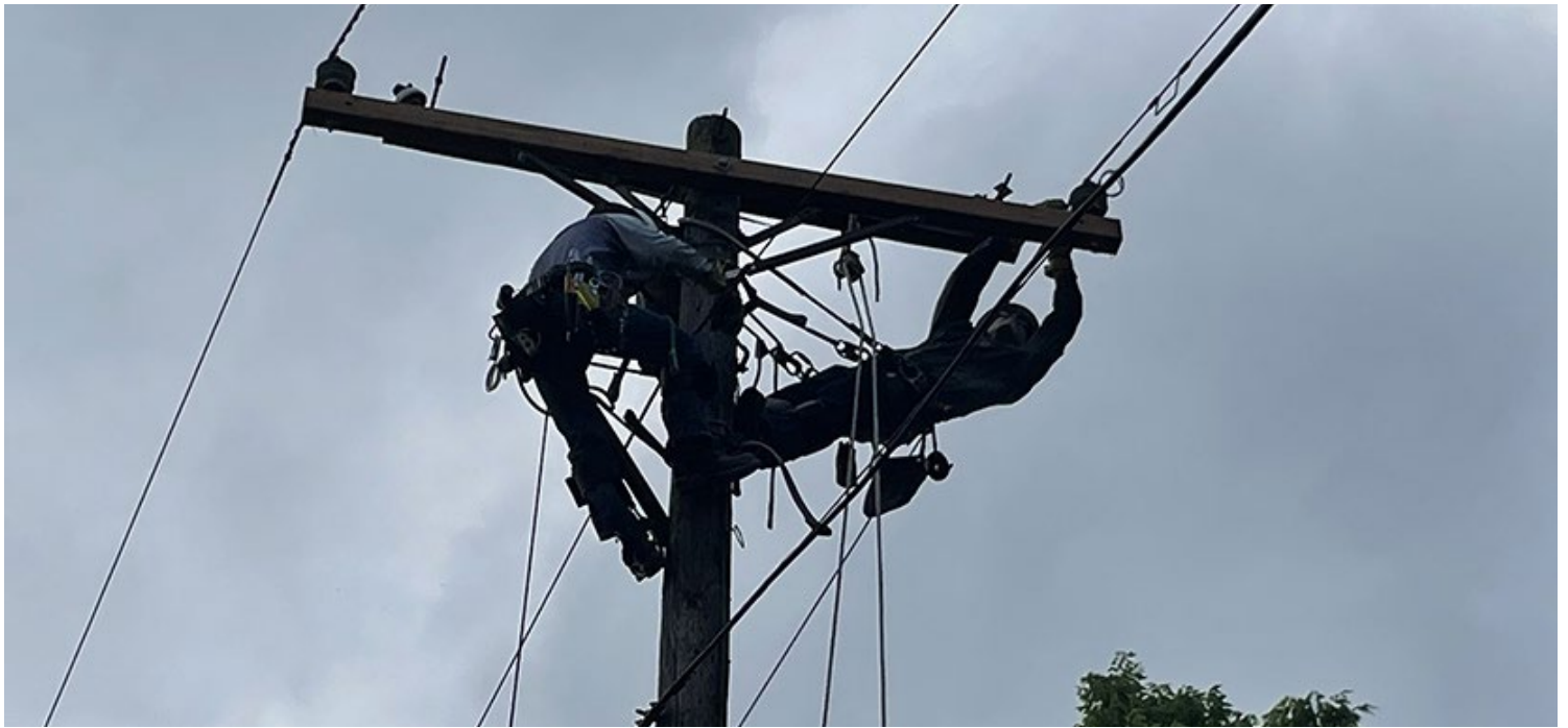
AEP Ohio linemen work to restore power. | AEP
