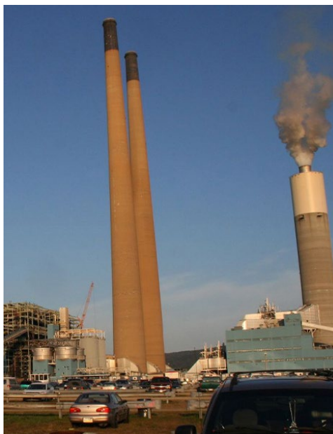
Conemaugh Generation Station | Dj245, CC BY-SA 3.0, via Wikimedia Commons
