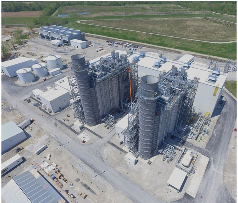
AES Indiana's 671-MW Eagle Valley combined-cycle gas turbine power plant in Martinsville, Ind., opened in 2018. The plant has since encountered technical issues and has been on an outage for more than a year. | AES Indiana
