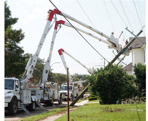
Utility workers restore downed power lines in Louisiana following last year's Hurricane Ida. | Entergy
