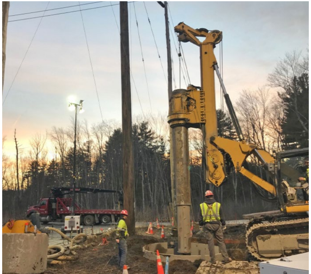
Construction of 345-kV transmission line foundations | Michels Power
