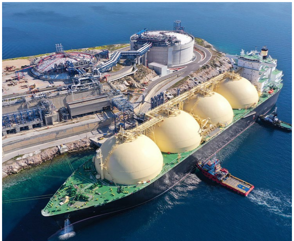
Energy experts say that global natural gas demand could allow the U.S. to displace gas from its power market for liquefaction and exportation. | Shutterstock
