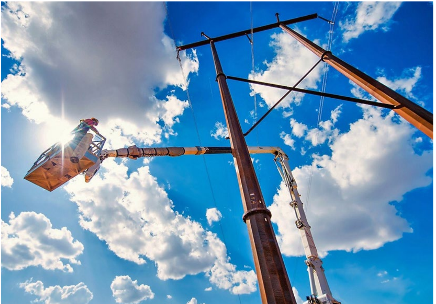
Xcel Energy lineman at a transmission tower | Xcel Energy
