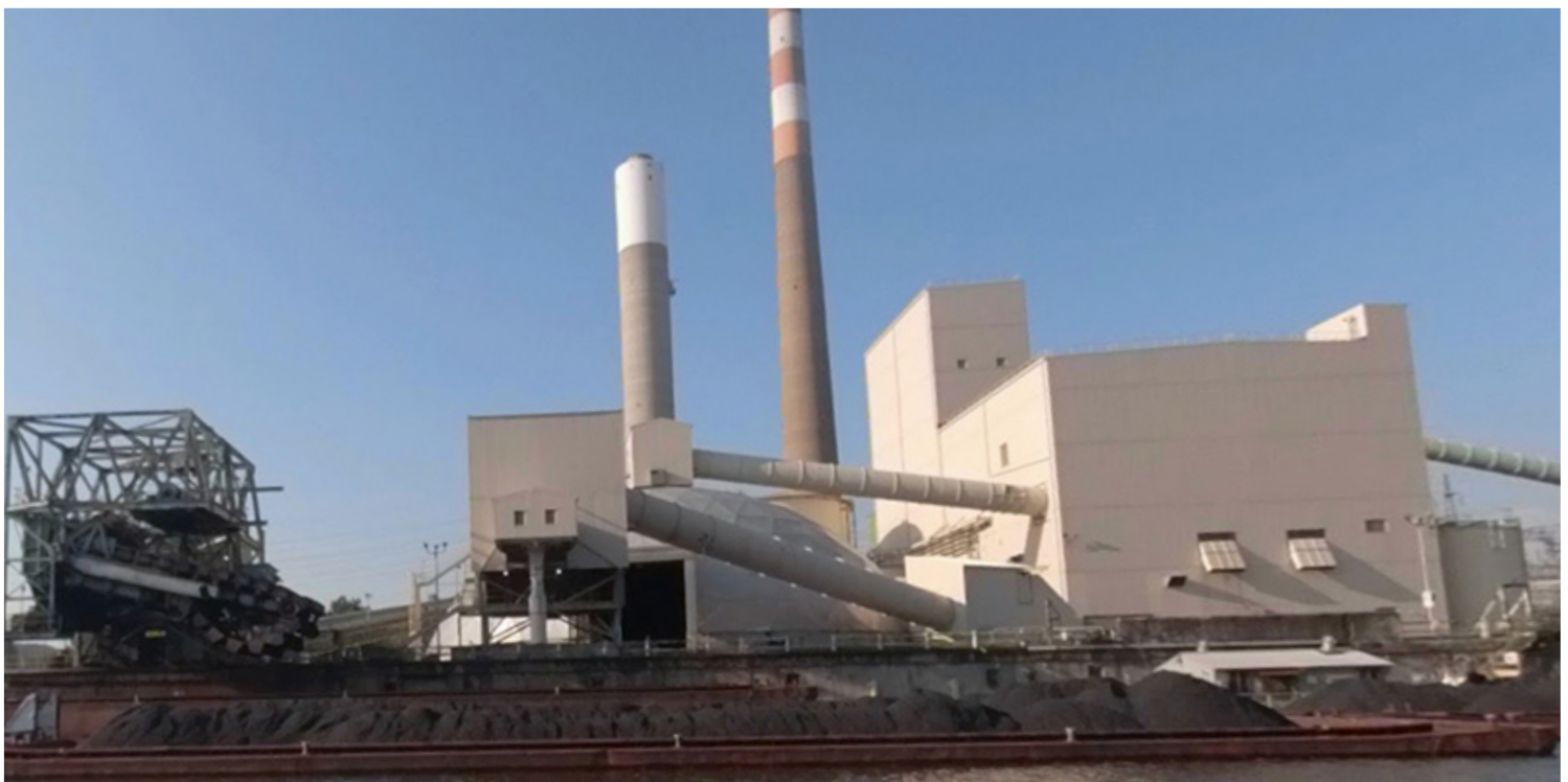
The coal-fired Cheswick generating plant in Springdale, Pa., retired in March 2022. | Google
