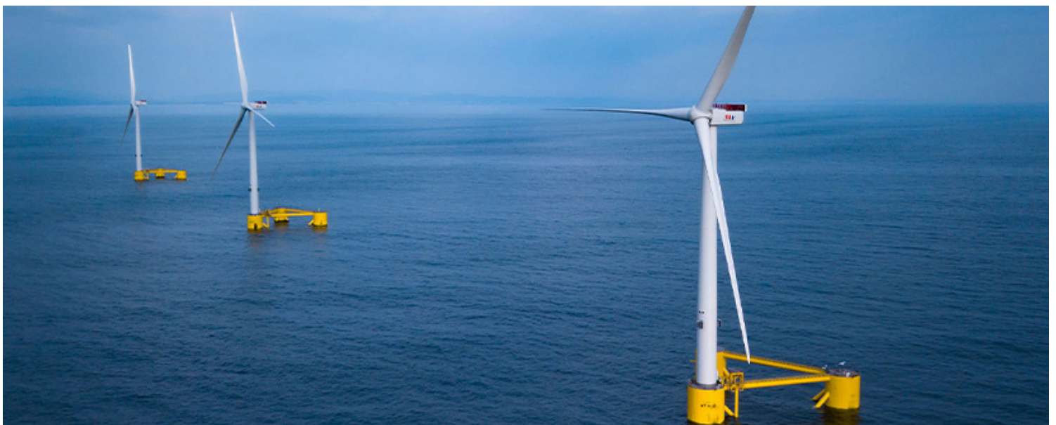
California will rely on floating turbines like those already being used in areas off the coast of Europe. | Principle Power
