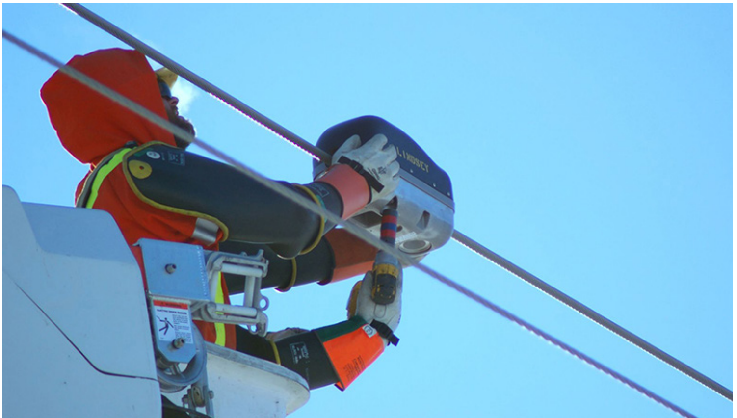
Installation of Lindsey SMARTLINE conductor monitor. | Lindsey Systems
