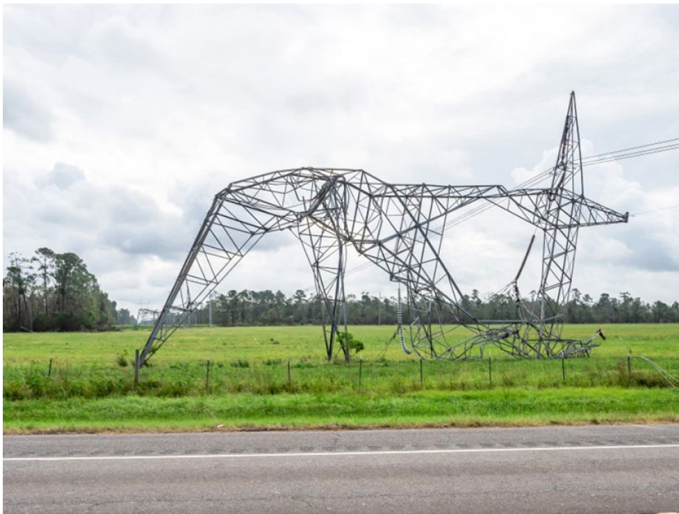
Damage to a Louisiana transmission tower from 2020's Hurricane Laura | Entergy
