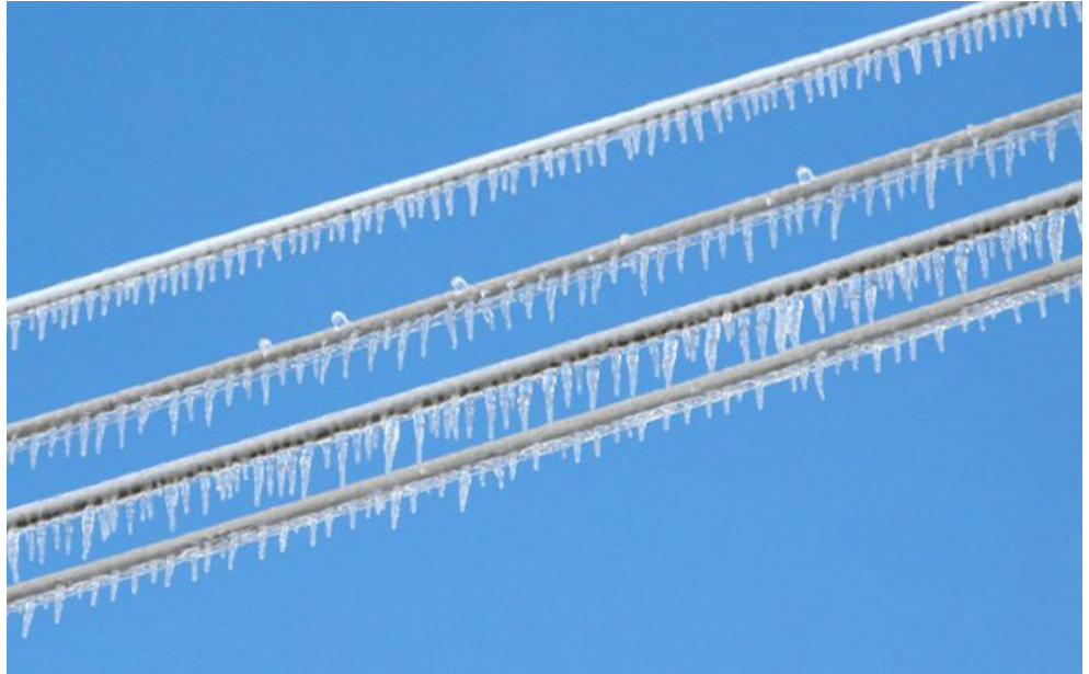
Ice hangs on power lines during the 2021 winter storm. | Energy
