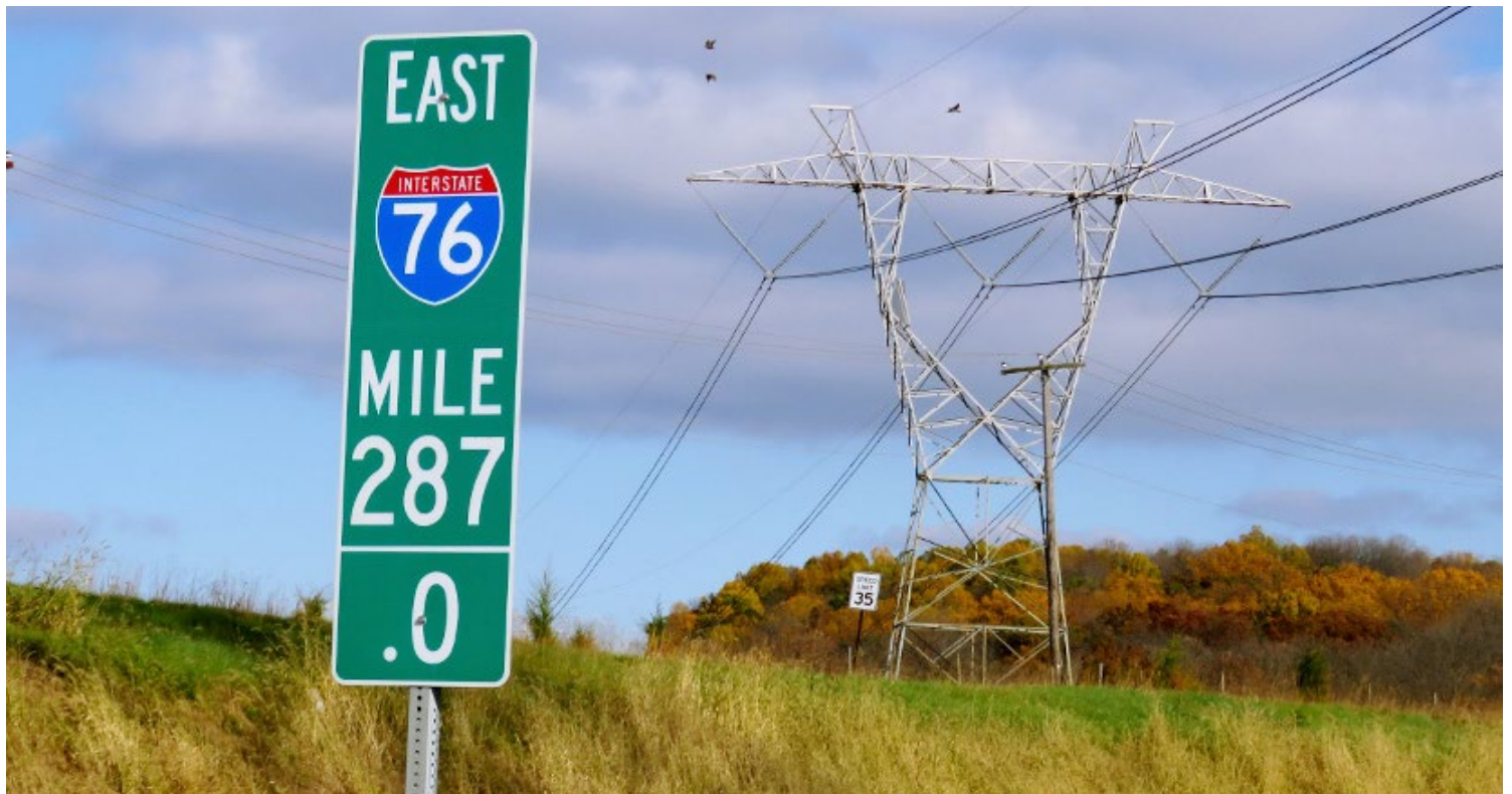
Transmission lines crossing the Pennsylvania Turnpike | © RTO Insider LLC
