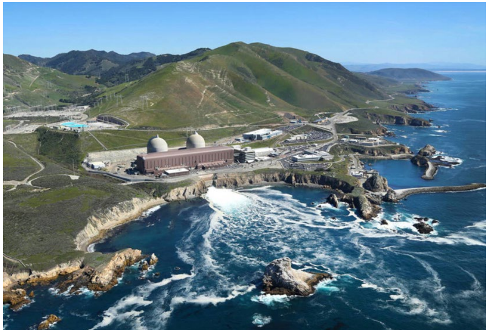
Diablo Canyon Power Plant sits on the coast of Central California. | PG&E
