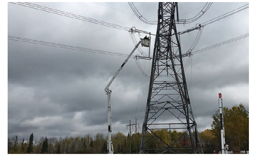
Xcel Energy line work in Northern Minnesota | Xcel Energy
