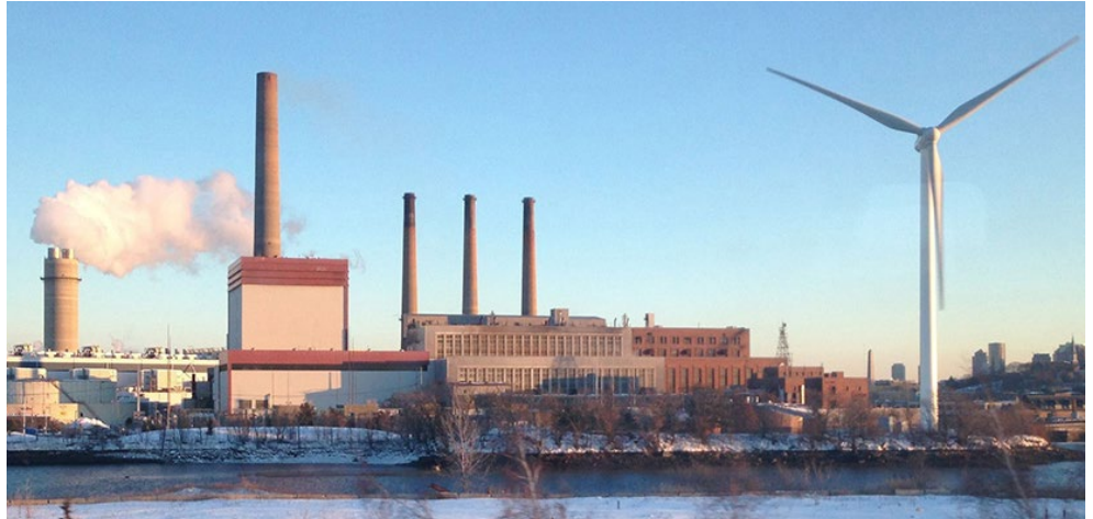
Mystic Generating Station is at the heart of debates around natural gas and grid reliability in New England. | Fletcher6, CC BY-SA 3.0, via Wikimedia Commons
