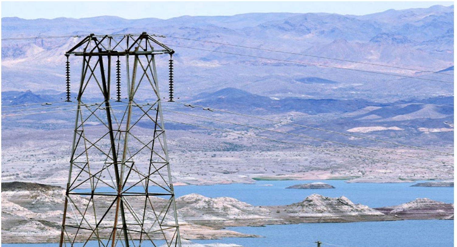
Transmission line near Lake Mead in Nevada. | © RTO Insider LLC
