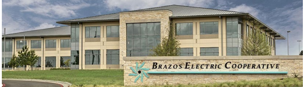
Brazos Electric has been given the go-ahead to solicit votes for its bankruptcy-exit plan and settle its dispute with ERCOT. | White Construction Co.
