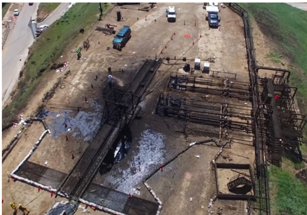
The SS-25 well at Aliso Canyon spewed 107,000 tons of natural gas over four months. | Blade Energy Partners/CPUC
