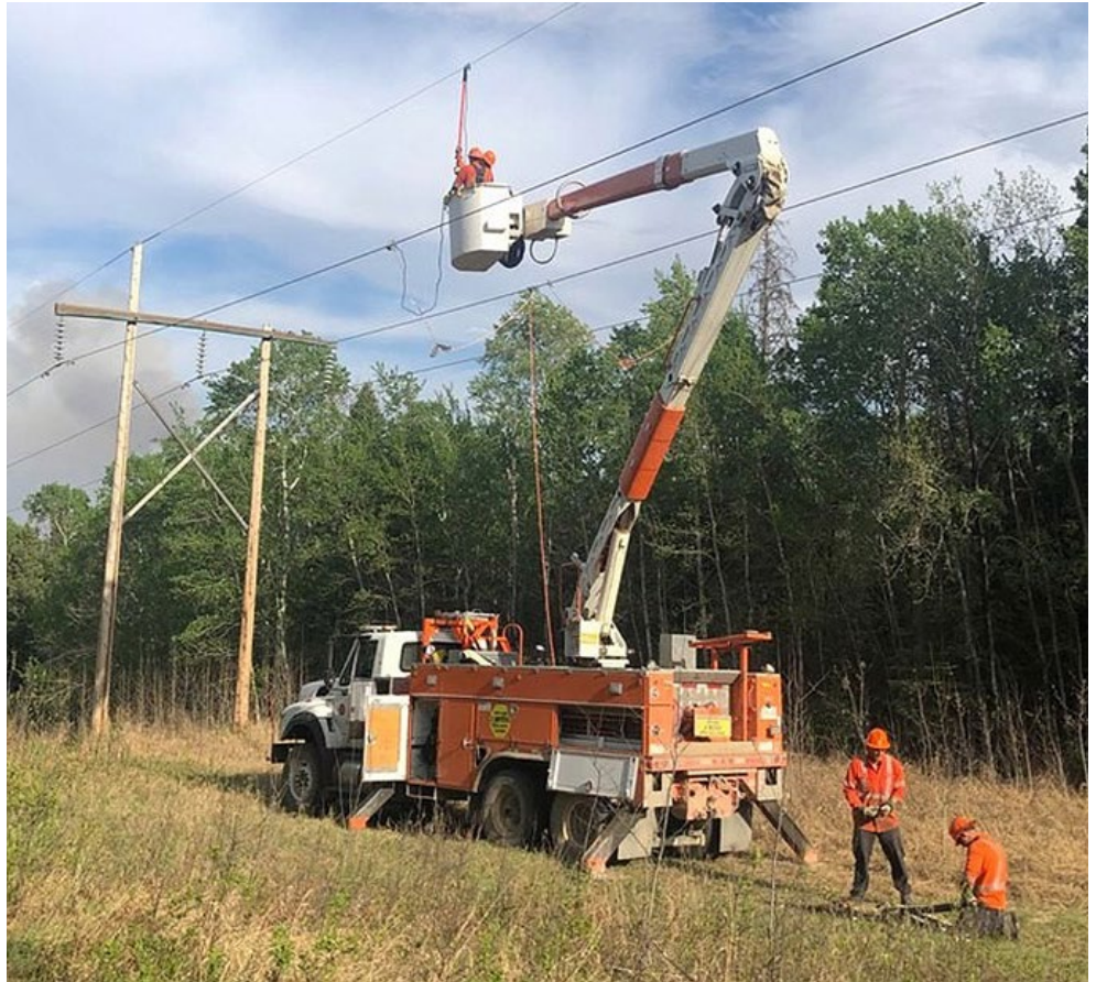
SaskPower line crew at work | SaskPower
