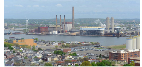
The Mystic Generating Station remains at the center of conversations about reliability and cost in New England. | Shutterstock
