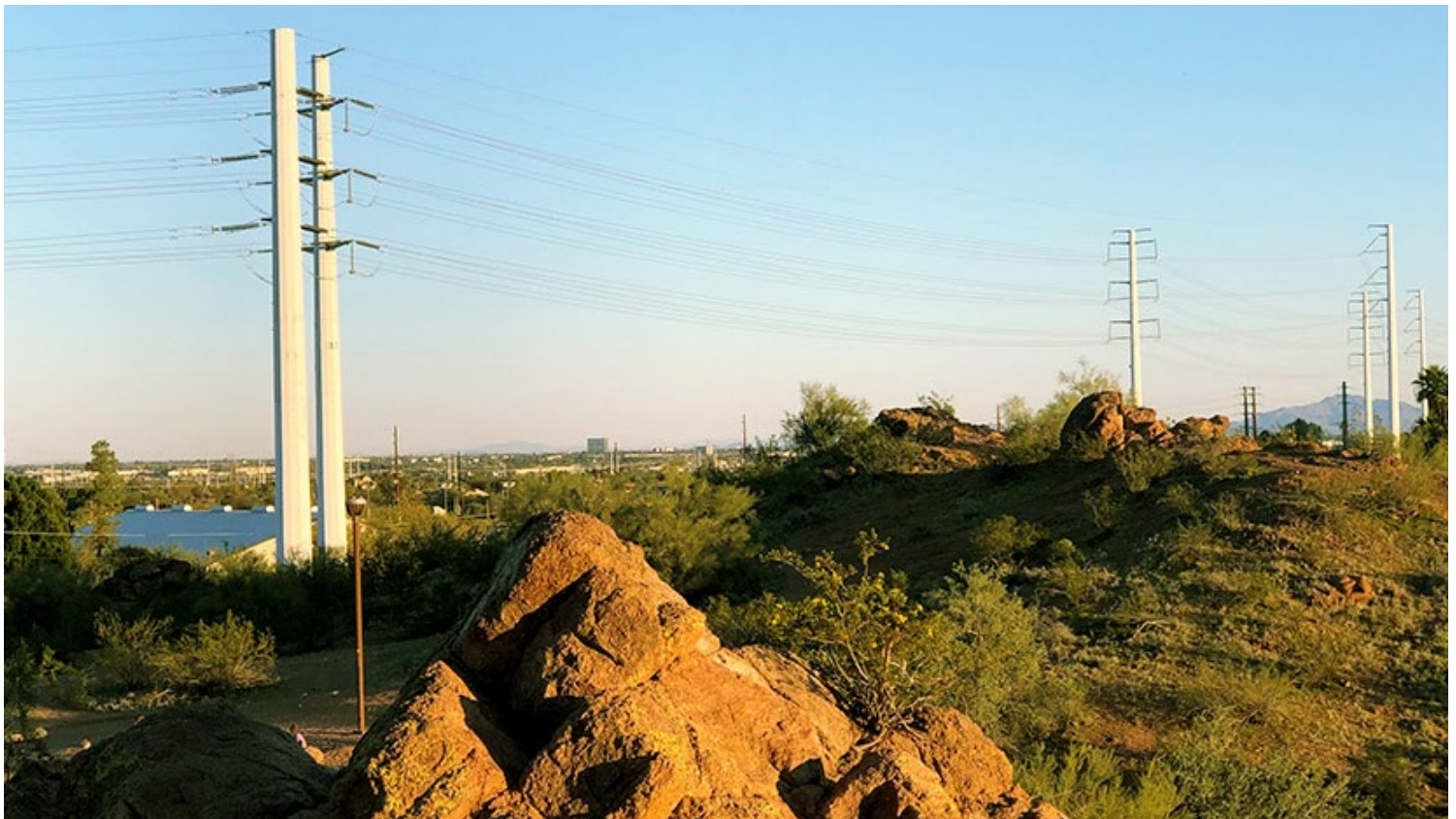
A power line crosses Tempe, Ariz., where WMEG members spoke at the fall CREPC-WIRAB meeting. | © RTO Insider LLC
