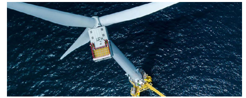
Wind power off the coast of California will require floating platforms because of ocean depths. | Principle Power
