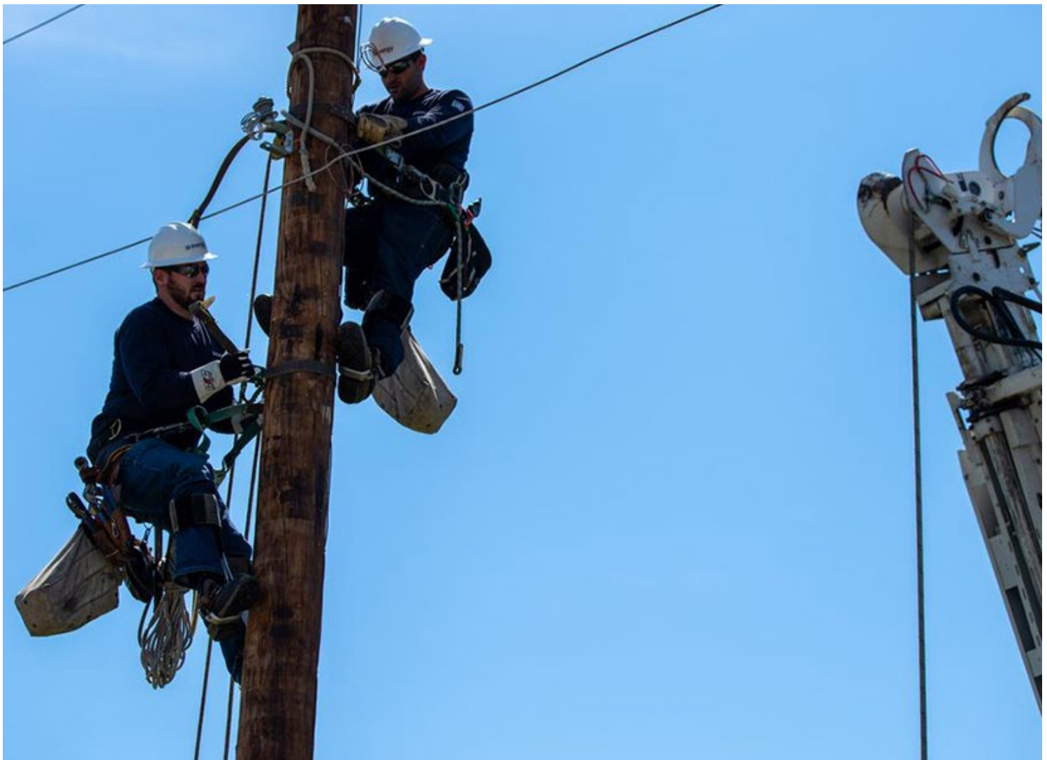
Evergy line crew at work | Evergy
