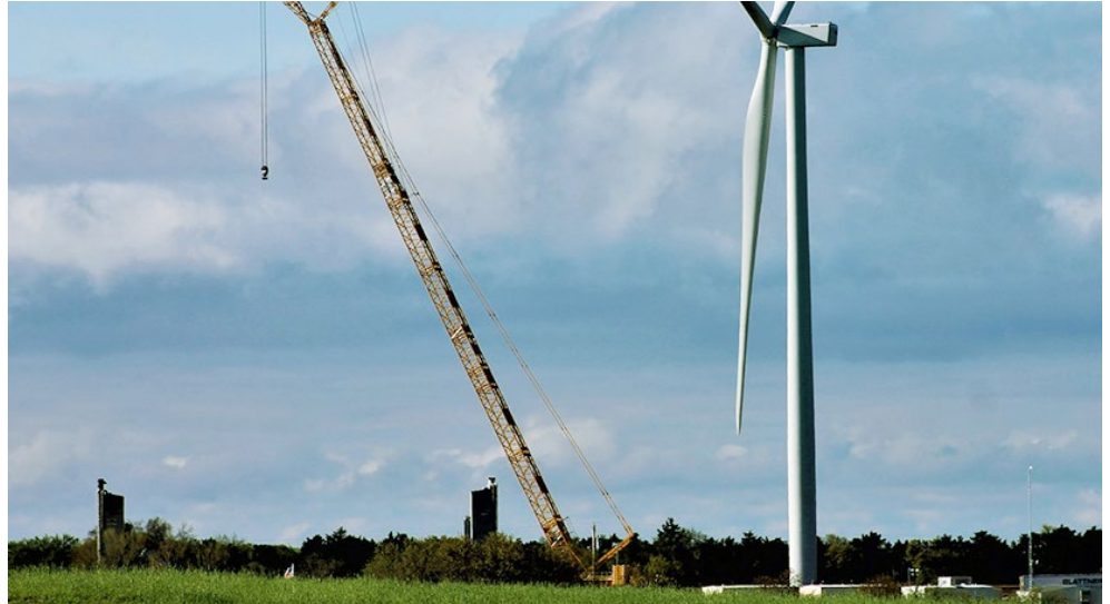
Turbine assembly at the 288-MW Maverick Energy Center in Oklahoma | Invenergy
