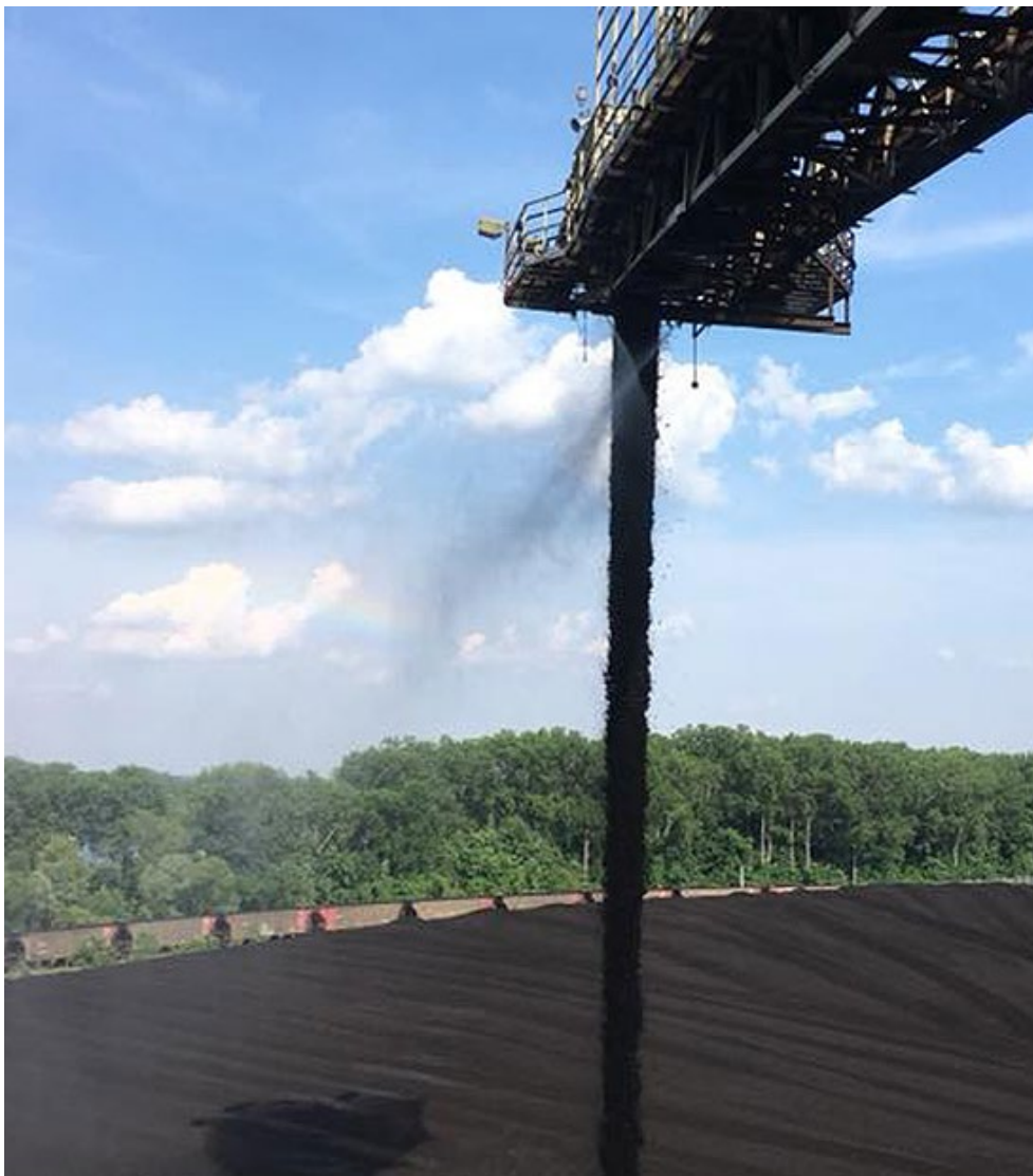
Coal coming off a stacker at Ameren Missouri's Rush Island plant in 2018 | Power Techniques Inc.
