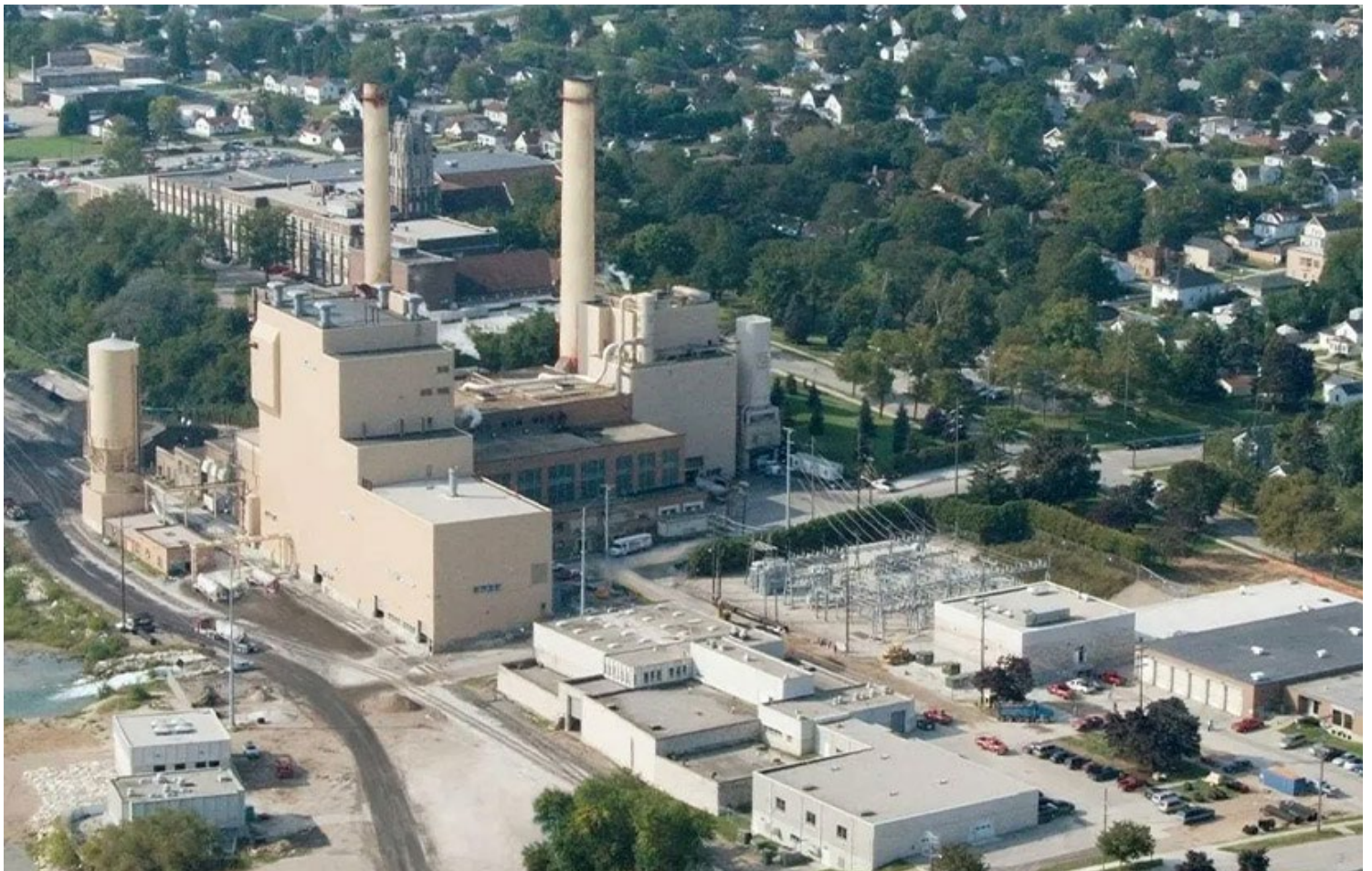
Manitowoc Public Utilities' Lakefront power plant | Manitowoc Public Utilities
