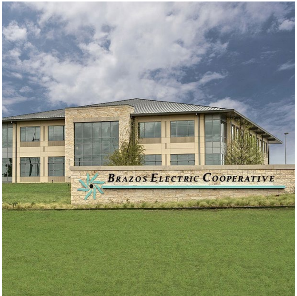
ERCOT and Brazos Electric Cooperative have settled their bankruptcy disagreements. | White Construction Co.
