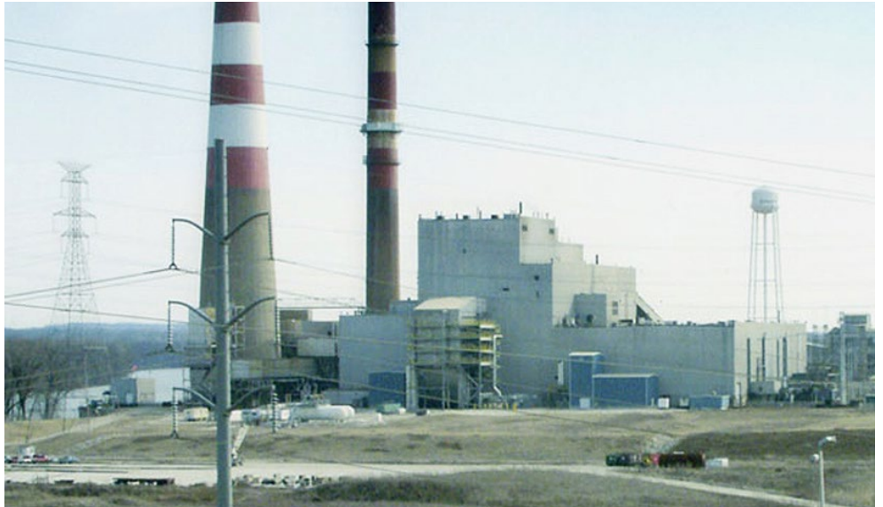
Edwards Power Plant | Sierra Club
