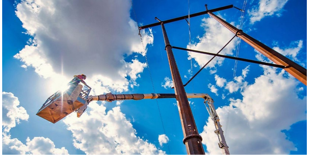
Xcel lineman works on upgrades to a transmission line. | Xcel Energy
