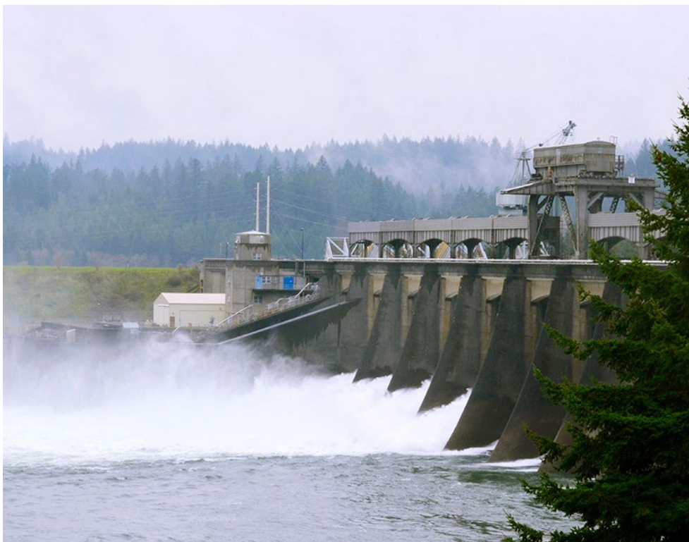
Spillway structure at BPA's Bonneville Dam | © RTO Insider LLC
