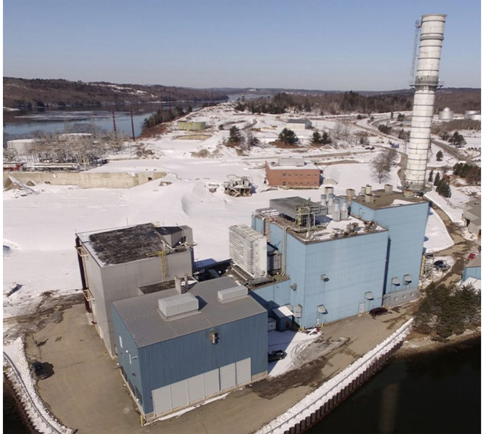
The Bucksport power station, one of the units involved in the deal | JERA
