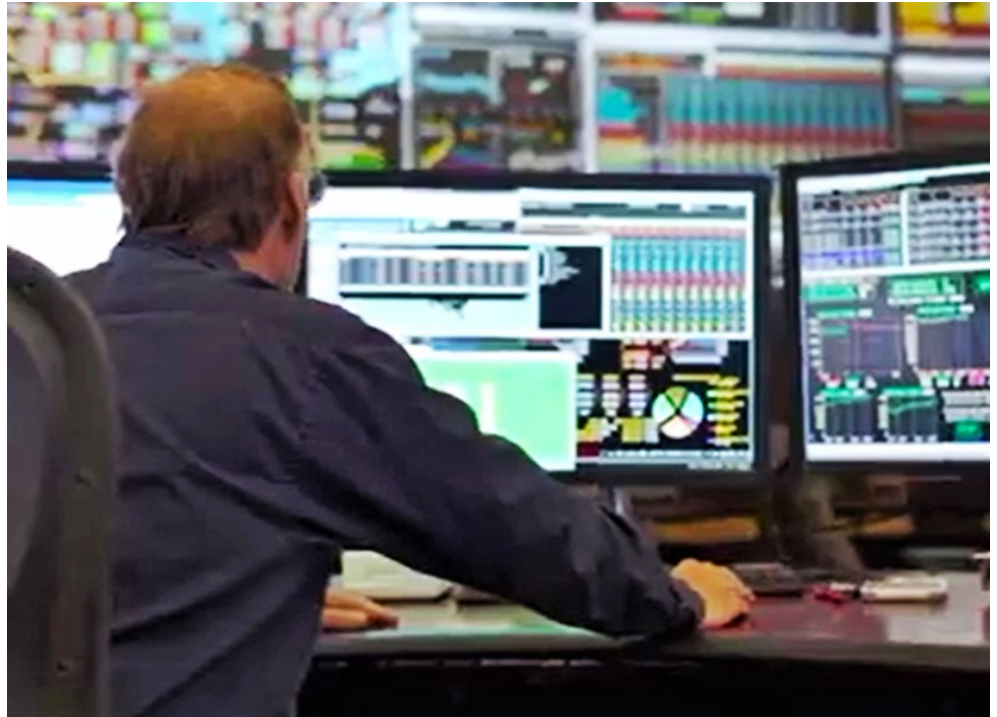
MISO operator manning control room | MISO
