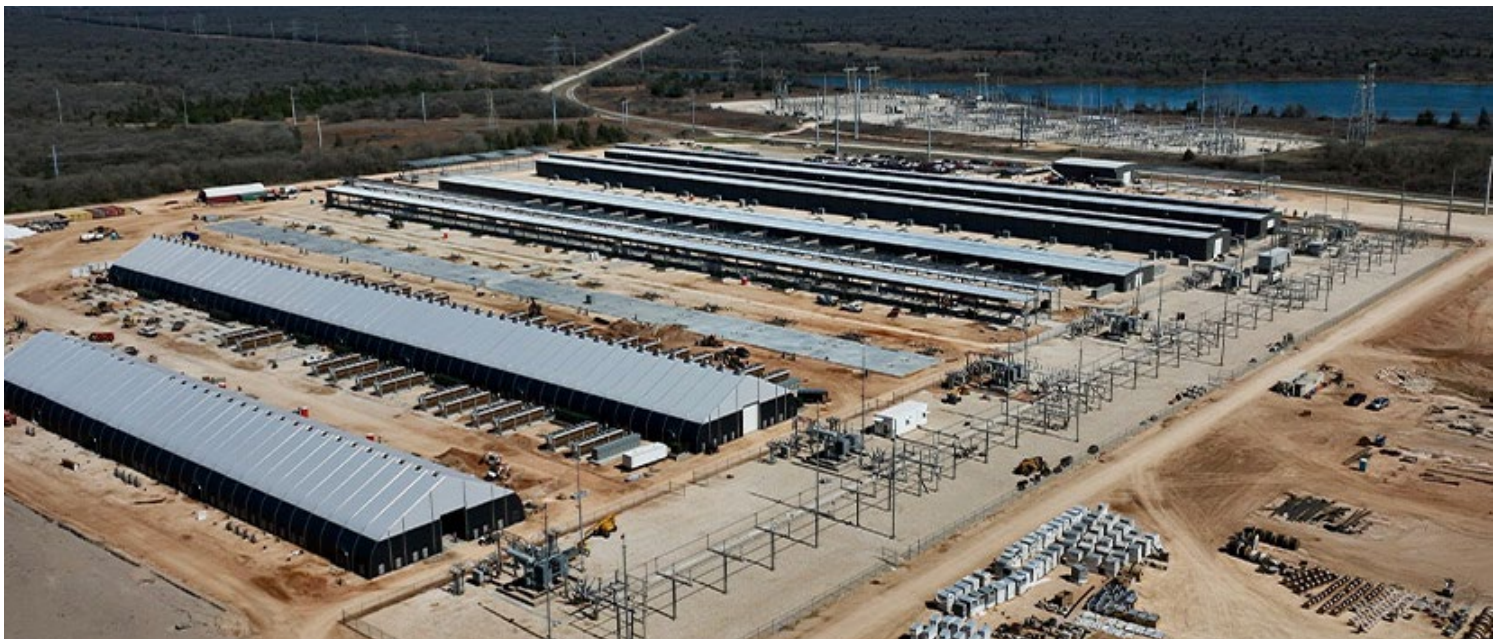
Bitcoin mining facility in Rockdale, Texas. | Riot Blockchain
