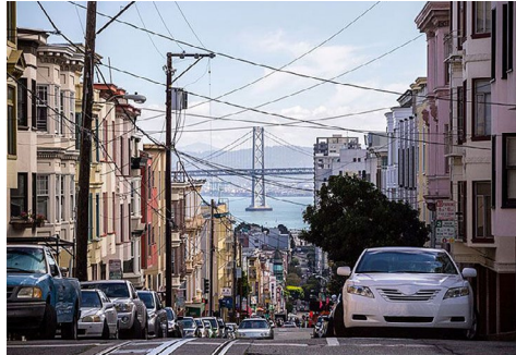
Distribution lines in San Francisco. | Contractors Insurance Agency
