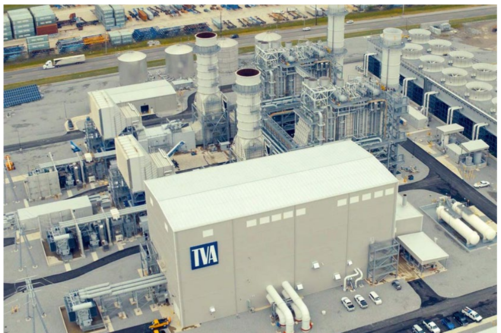
TVA's Allen Combined Cycle Plant near Memphis, Tenn. | TVA
