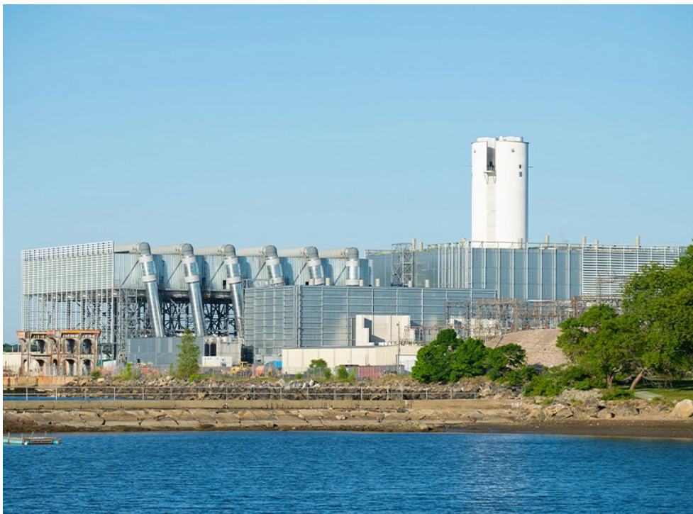
Salem Harbor Power Station, a gas-fired generating plant in Salem, Mass. | Fletcher, CC BY-SA 4.0, via Wikimedia Commons
