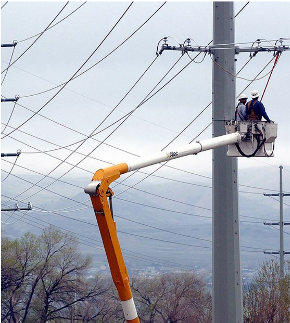
Lineworkers on a PacifiCorp transmission line | PacifiCorp
