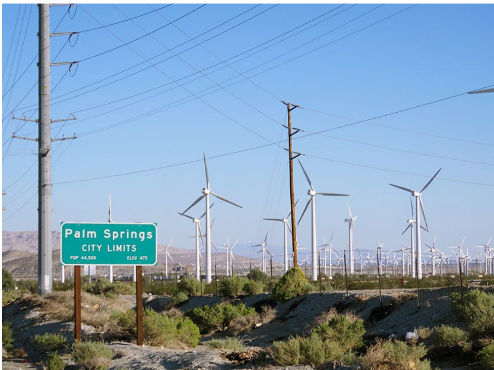
Wind farm near Palm Springs, Calif. | © RTO Insider LLC
